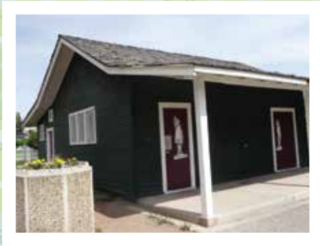
{ Elbow River building } 2011 | The City of Calgary Parks
