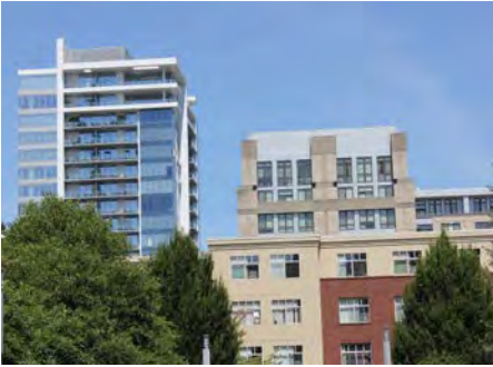
A mix of quality buildings of varying forms and heights supports attractive and vibrant urban areas.
