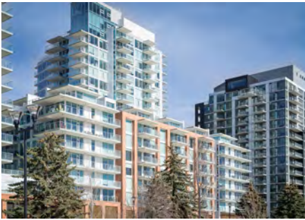
Variation in building massing in East Village.
