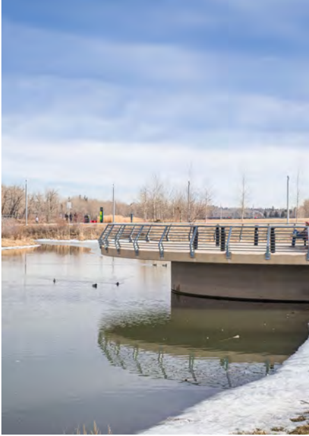
Stormwater pond in East Village.
