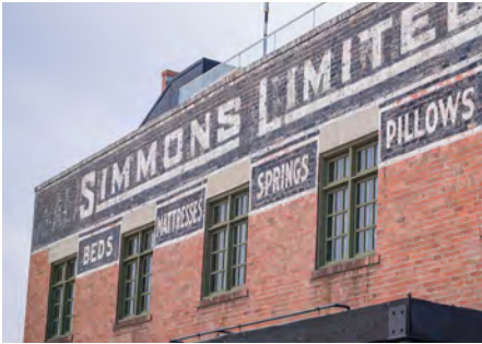
Simmons building in East Village.
