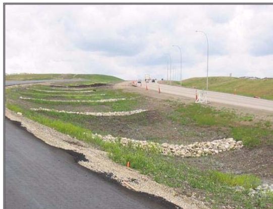
Figure 9-13: Rock Check Dam
