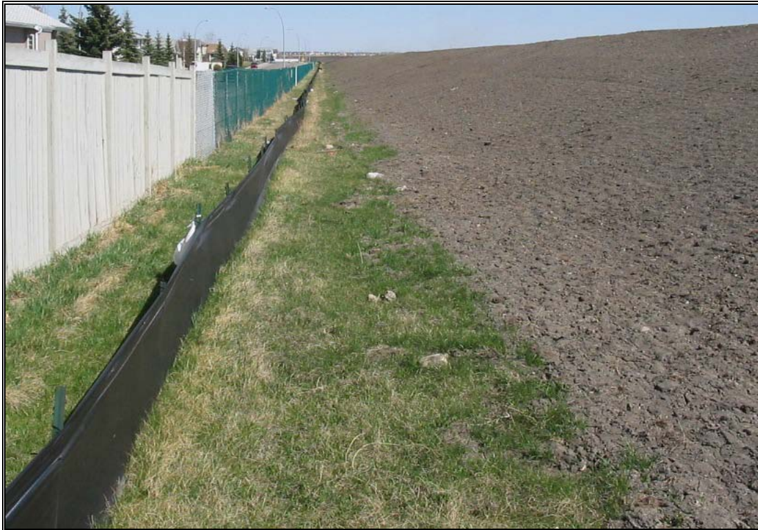
Photo 1: Use of a vegetated buffer strip in combination with a perimeter silt fence and a topsoiled and tracked slope. BMPs work most effectively if they are implemented as part of a system of erosion & sediment control.
