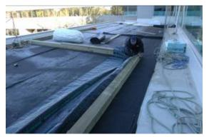
(e) Installation of root barrier
