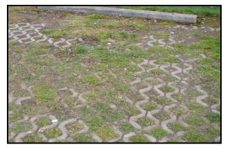
Figure 5-24 Improperly Installed Turf Paving Stone System
