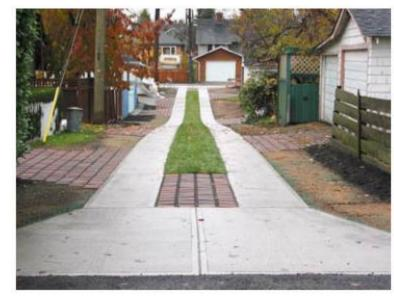
Figure 1-6 Example of water sensitive alley
