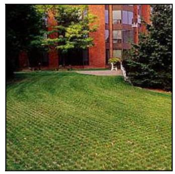
Figure 5-4 Turf Pavers planted with grass
