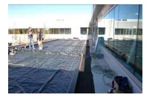
(f) Installation of Root Barrier
