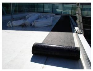
(a) Installation of drainage board
