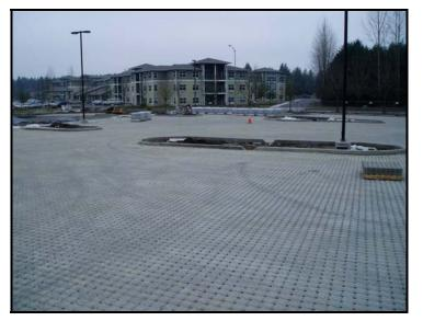
Figure 5-3 Permeable Unit Pavers at Parking Lot in Olympia, Washington
