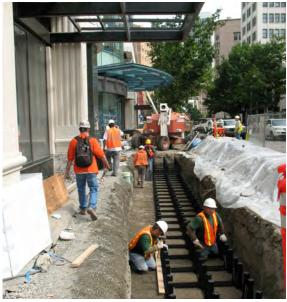
This modular structure for tree boulevards should prevent damage of adjacent pavement and underground utilities by spreading roots and will provide predictability for future nearby work under the pavement.
