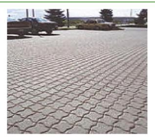
Figure 8: Enlarged Permeable Joints
