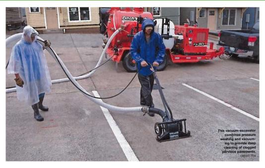
Figure 12: Pressure Vacuum and Washing Equipment (Courtesy of Concrete Construction June 2013)
