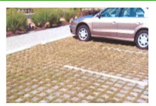
Figure 10: Concrete Grid Porous Pavers
