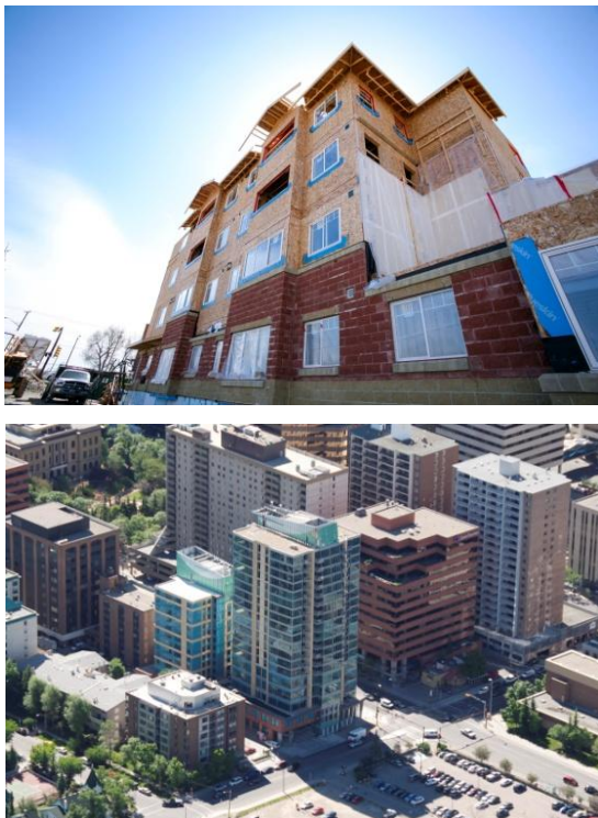
Figure 13: (Top) Crestwood (wood frame) and (below) Louise Station (concrete).
