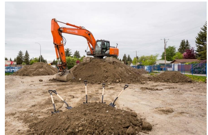
Figure 10: Wildwood affordable housing development ground breaking
