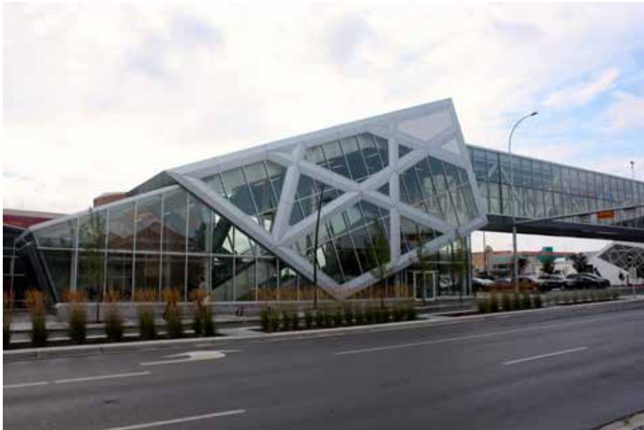
Figure 7 | 61 Avenue SW Pedestrian Bridge
