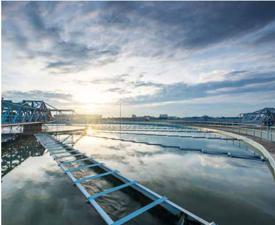
Figure 17 | Water treatment plant
