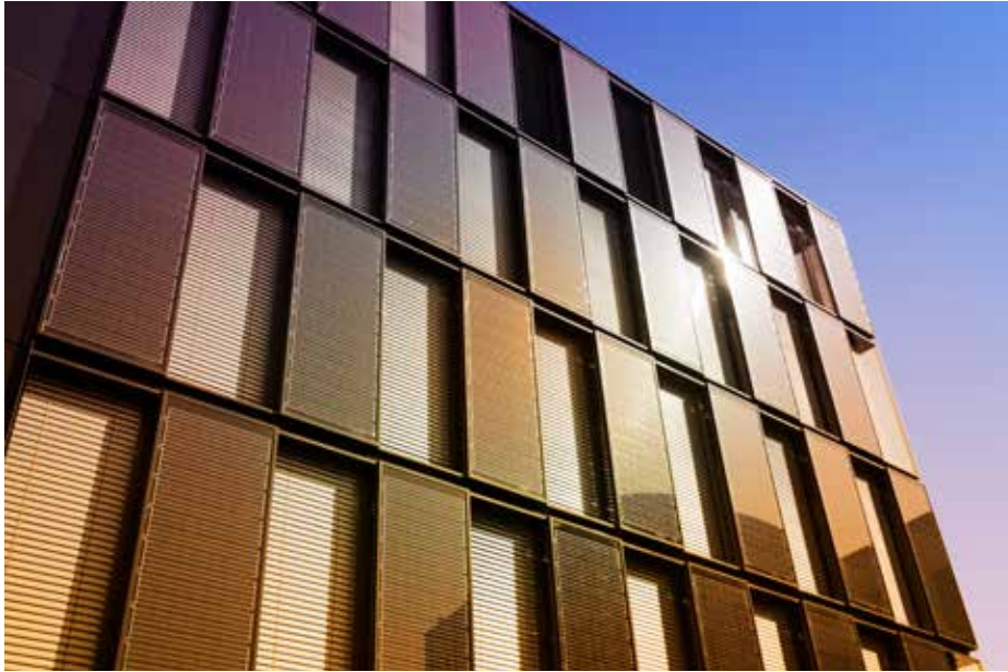
Figure 9 | Solar panels on building façade
