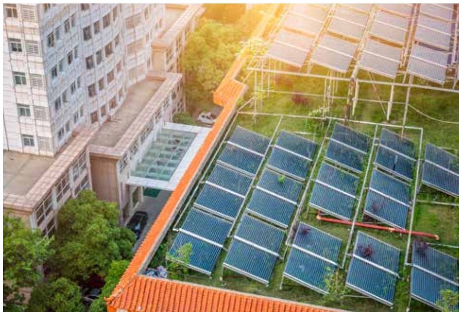
Figure 21 | Rooftop solar panels
