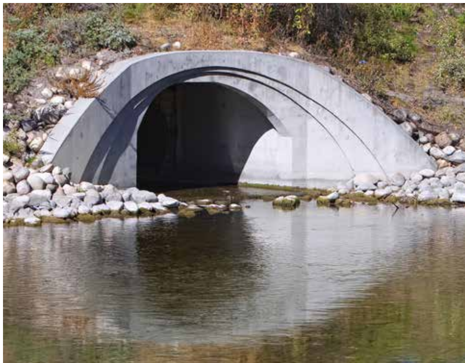
Figure 19 | Stormwater outfall
