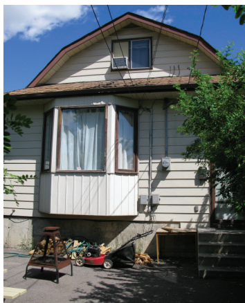
A resource with poor integrity
