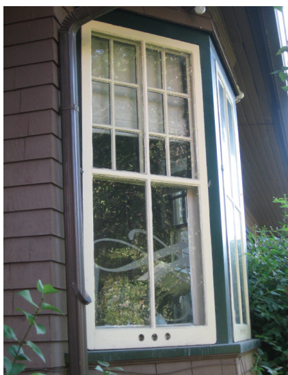
Window detail, Nellie McClung House (1907)
