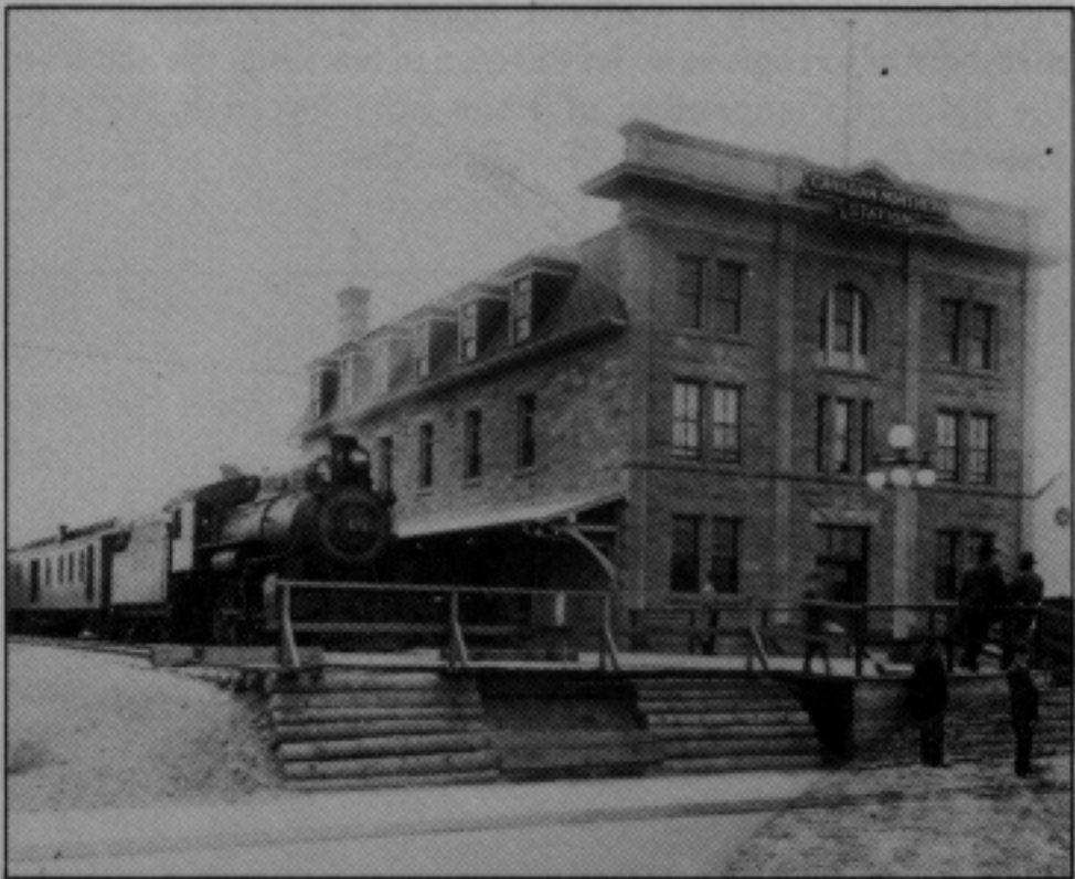
Canadian Northern Railway Station.
