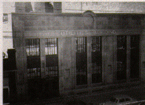
The Utilities Building, n.d. (CESA 8-14)
