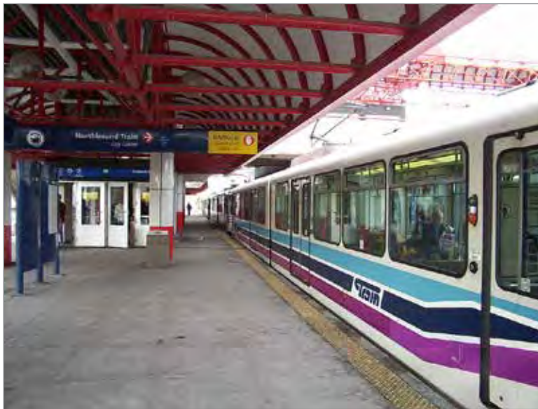
The south LRT station improvements will increase customer safety and comfort
