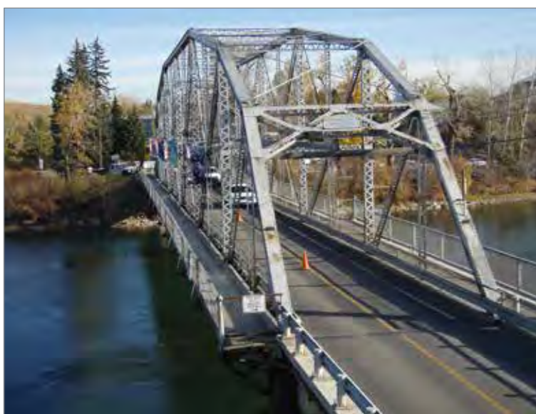
The 12 Street S.E. (Zoo) bridge accessing the Calgary Zoo will be replaced
