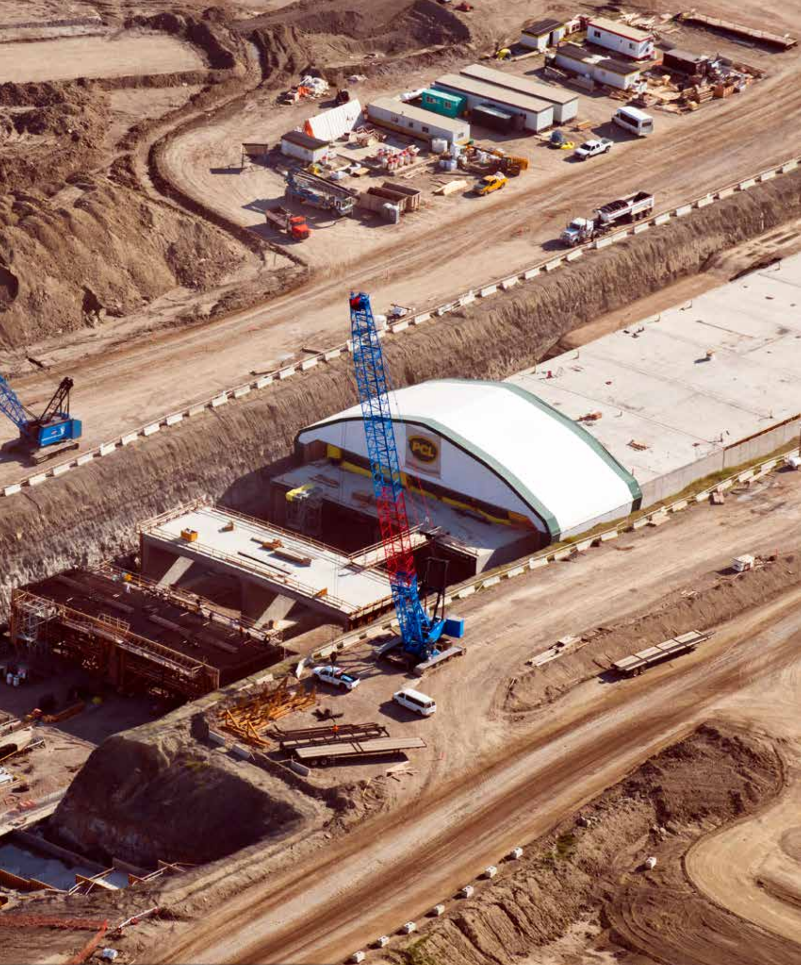
View of the Airport Tunnel - August 2011
