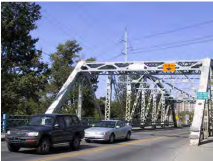
The 9 Avenue S.E. bridge spanning the Elbow River will be replaced
