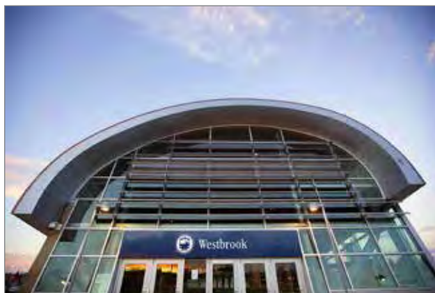
Westbrook CTrain station
