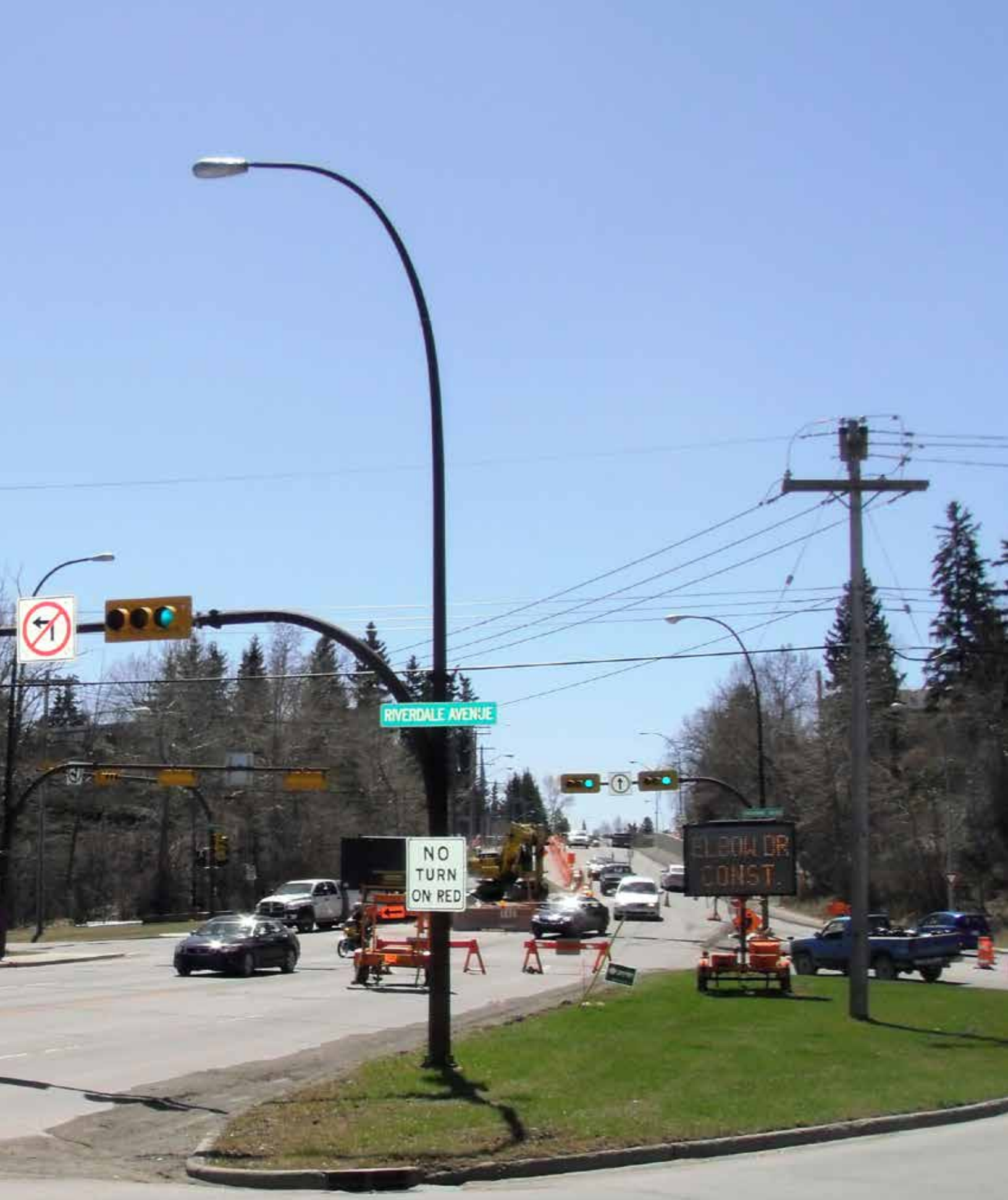
Elbow Drive Road Reconstruction - May 2011
