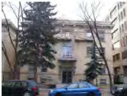
725 - 13 Avenue SW Houlton House (Congress) Apartments
