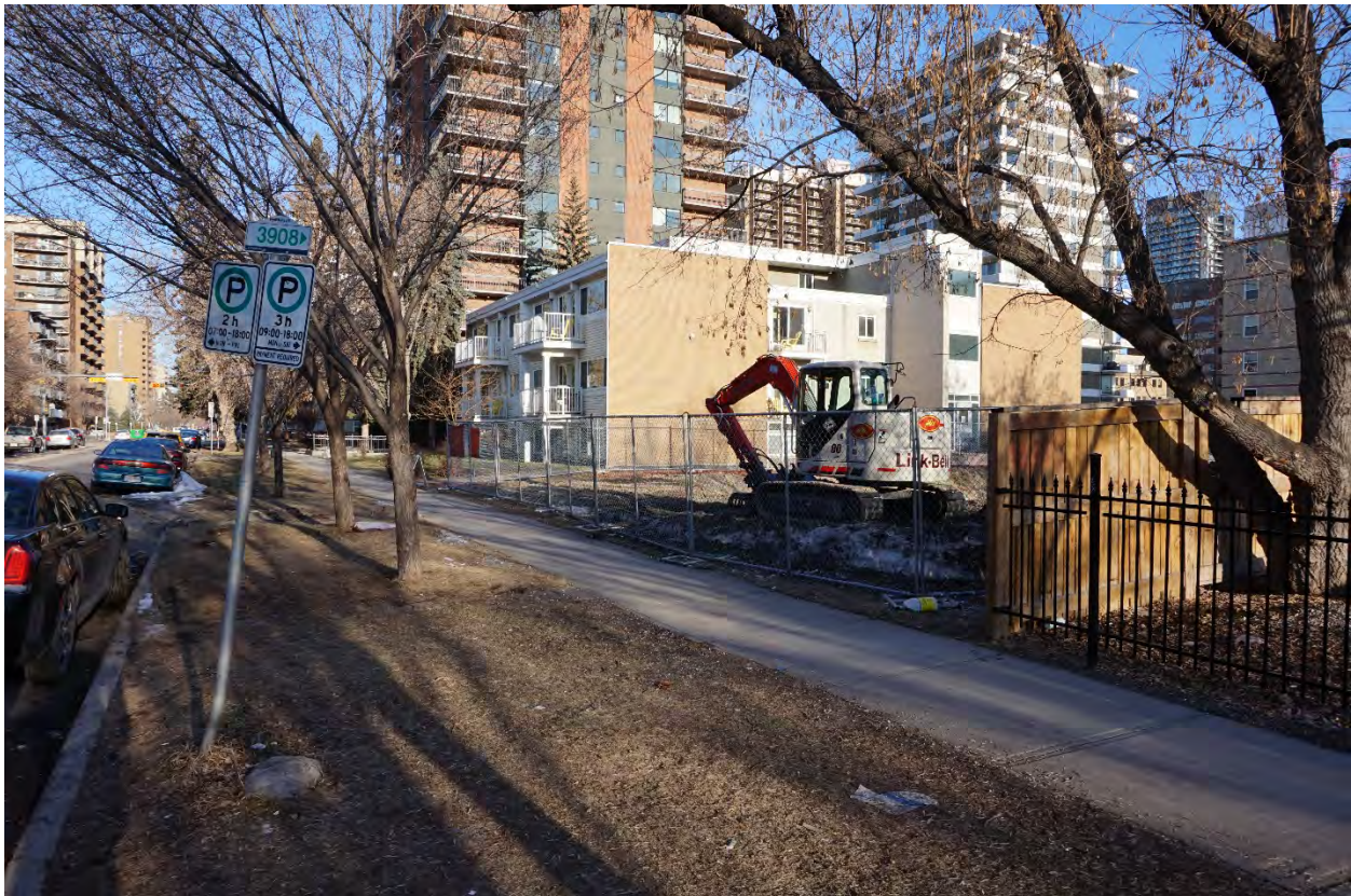
Receiving Parcel 1 (DC Site 1): 524, 528 and 536 - 14 Avenue SW
