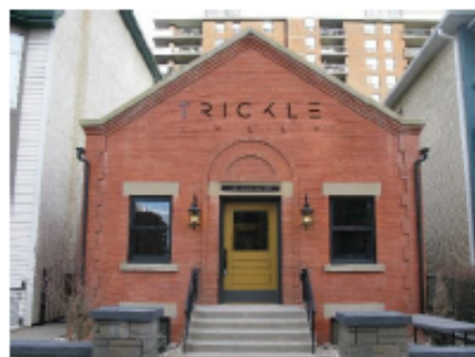
1010 - 14 Avenue SW West End Telephone Exchange
