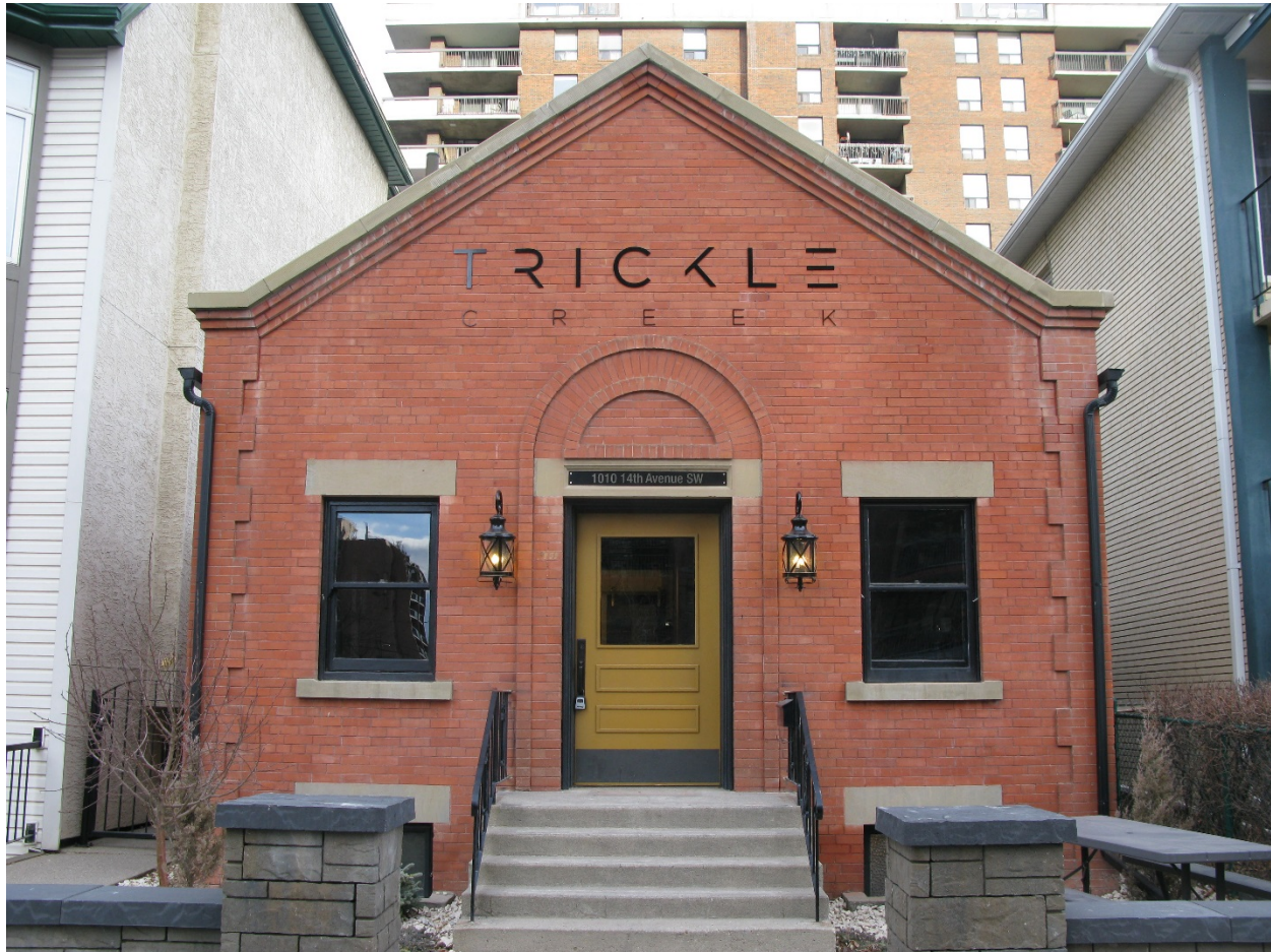
Source Parcel 3 (DC Site 5): 1010 - 14 Avenue SW - West End Telephone Exchange
