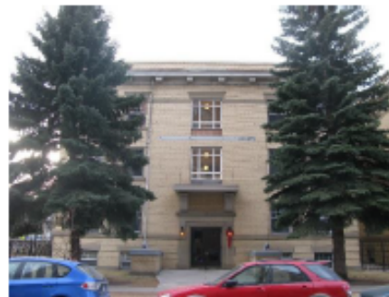
721 - 13 Avenue SW Moxam Apartments
