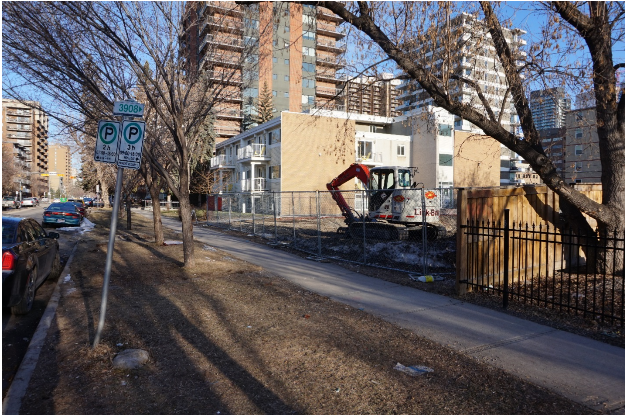
Receiving Parcel 1 (DC Site 1): 524, 528 and 536 - 14 Avenue SW
