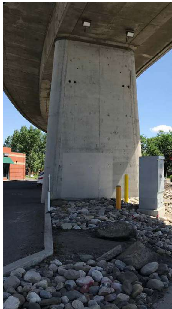
Existing flyover pillars
