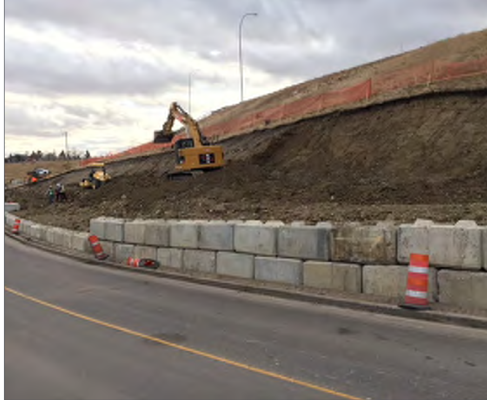
Retaining wall being built for new Bow Trail and 10 Avenue S.W. on-ramps
