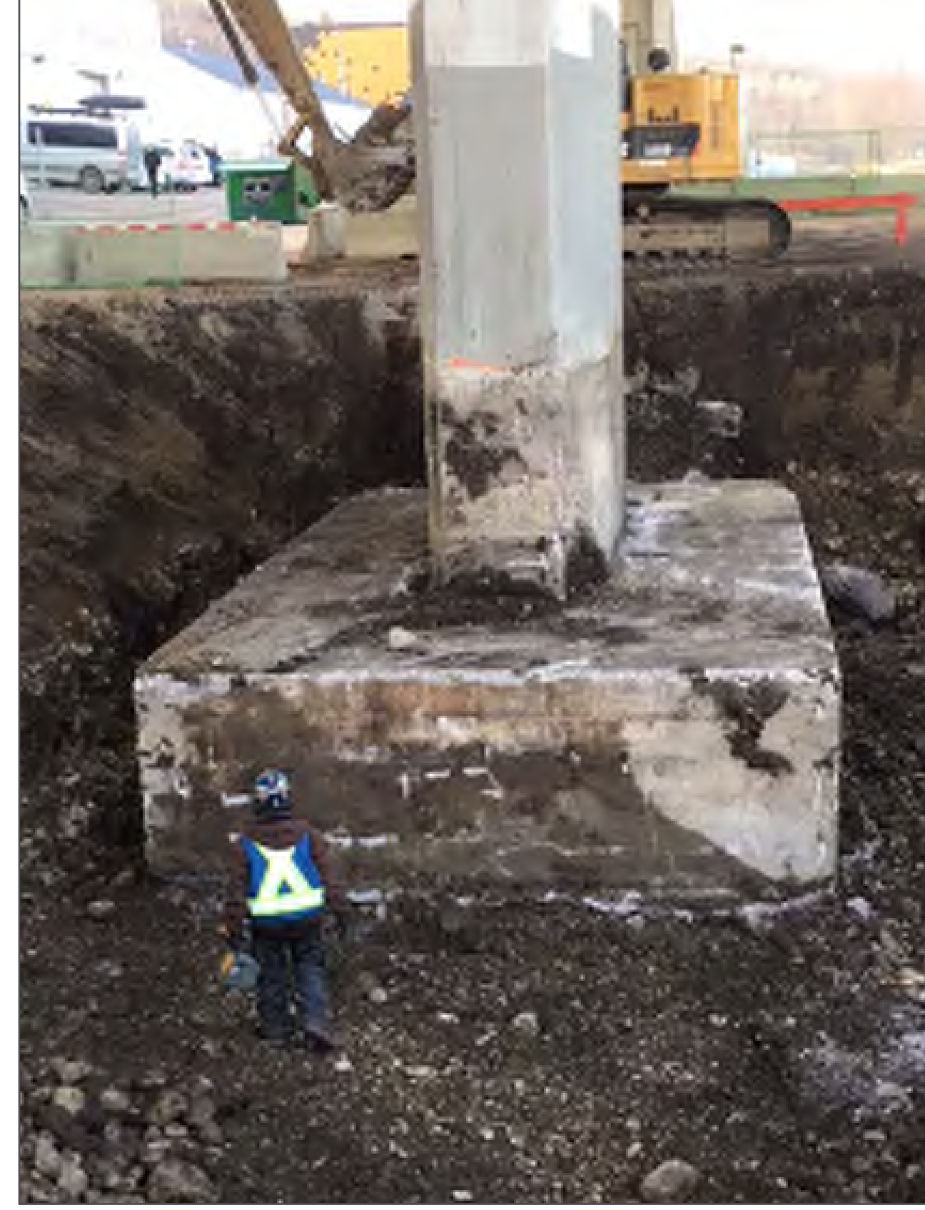
Widening and re-enforcing of the Bow River Bridge piers
