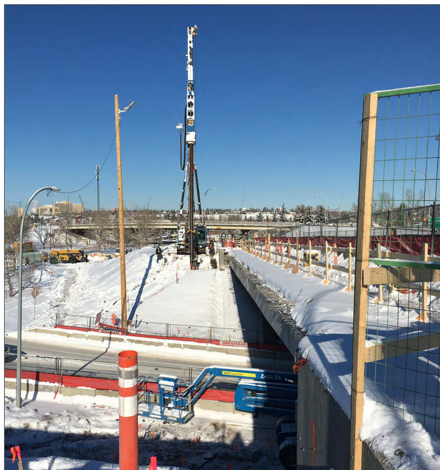
Widening of the bridge over Memorial Drive
