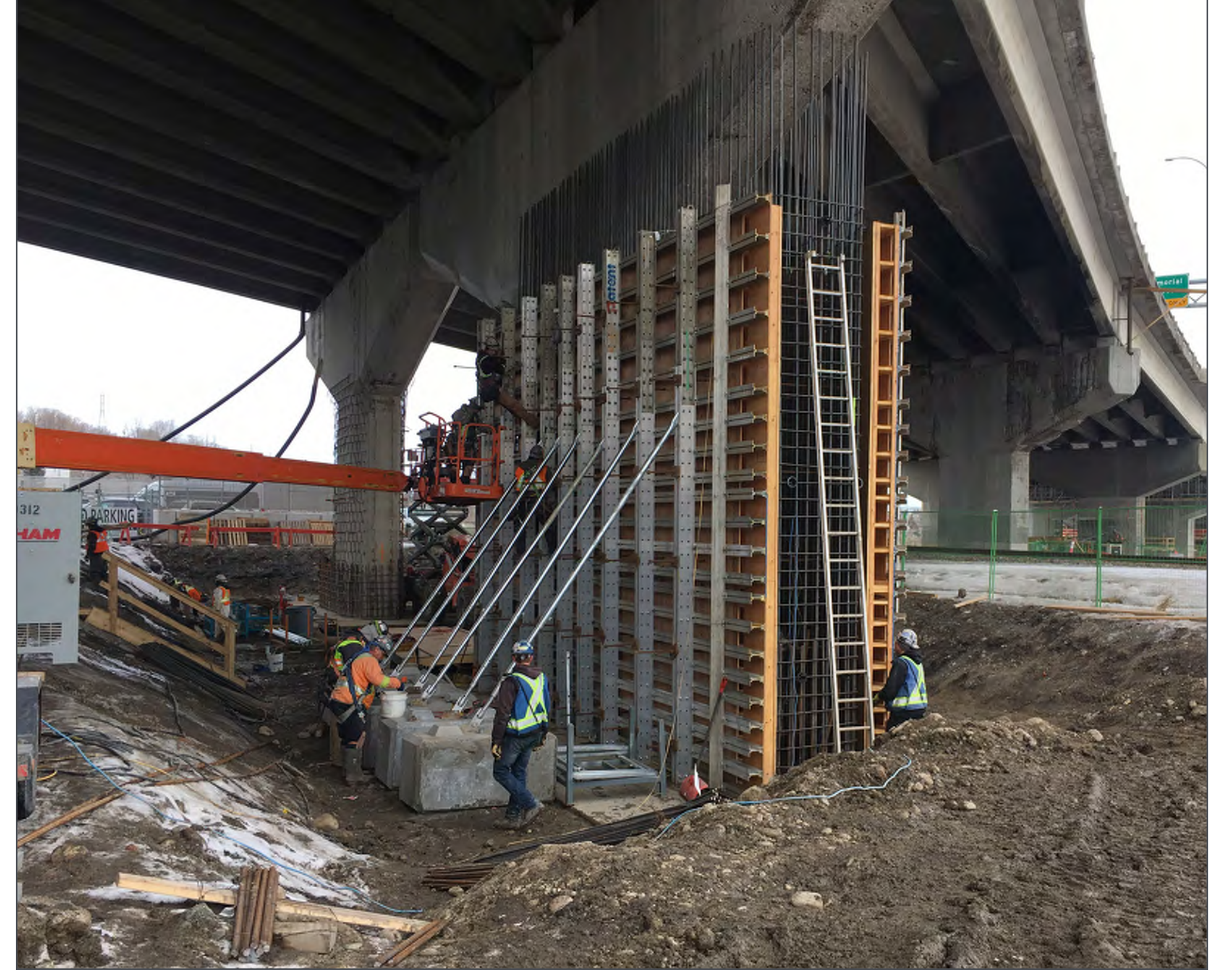
Widening and re-enforcing of the Bow River Bridge piers
