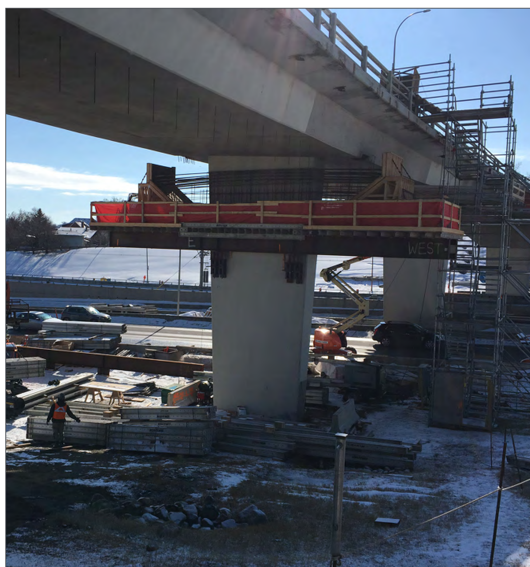
Widening of Bow Trail Bridge, including the installation of work platforms
