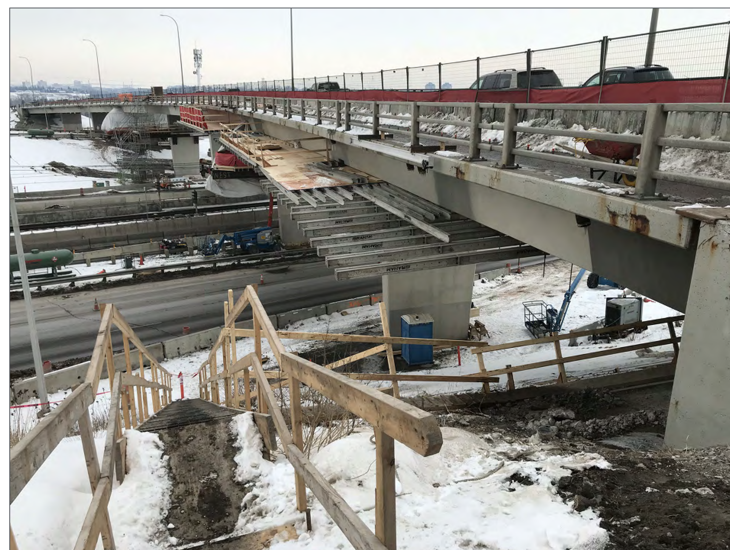
Widening of Bow Trail Bridge, including the installation of work platforms
