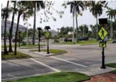
Figure 3.2-7: Rectangular rapid flash beacon
