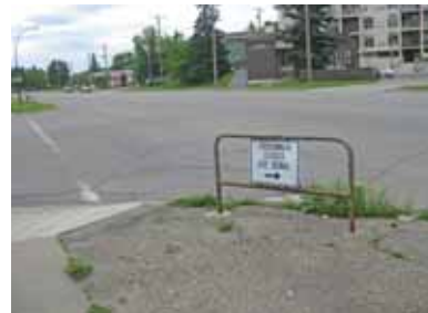
Figure 3.2-19: Closed crosswalk – 3rd Ave NW, Parkdale Community
