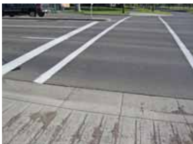
Figure 3.2-17: Advanced stop lines
