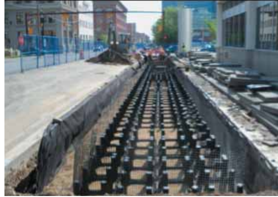
11 Avenue SW ENMAX Utility Line
