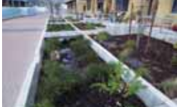
Penneyer Street, Portland
