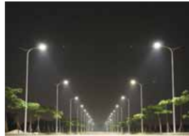
Figure 3.1-17: Travel way lighting
