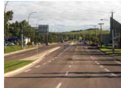
Figure 1.4-3: 106th Avenue S.E. adjacent to Southbend Business Park
