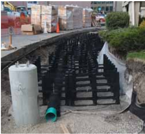
Figure 3.6-6: Soil Cell
