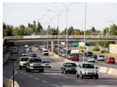
Figure 3.2-15: Pedestrian overpass on Crowchild Trail
