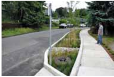
Figure 3.5-1 : Curb extension with rain garden
