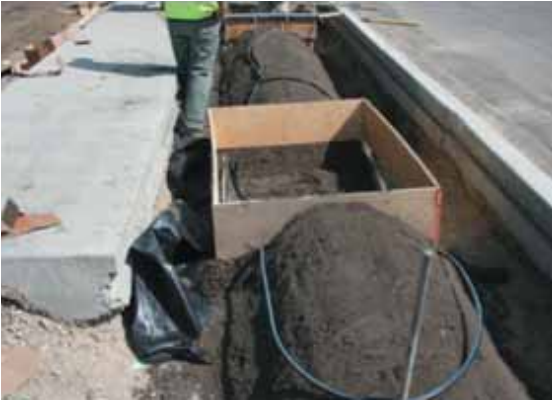
Tree trench during construction
