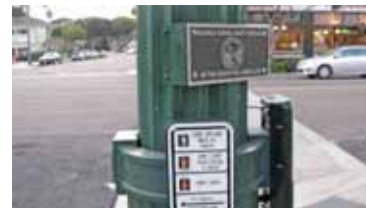
accessible pedestrian signals
