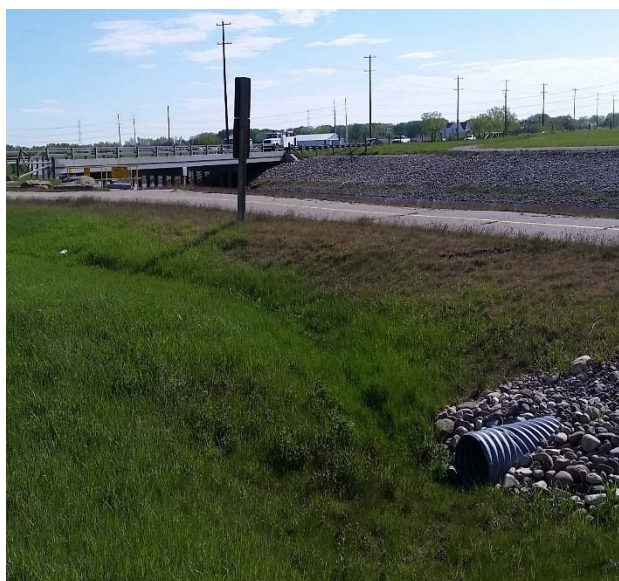
Figure 1.3: Southern canal culvert looking east
