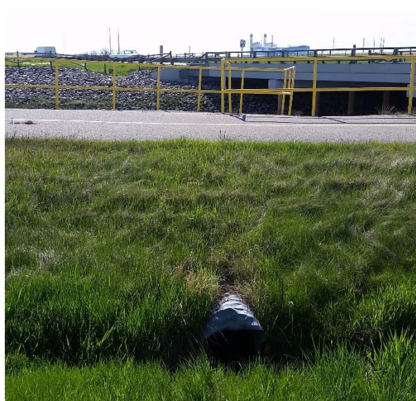
Figure 1.4: Northern canal culvert looking east
