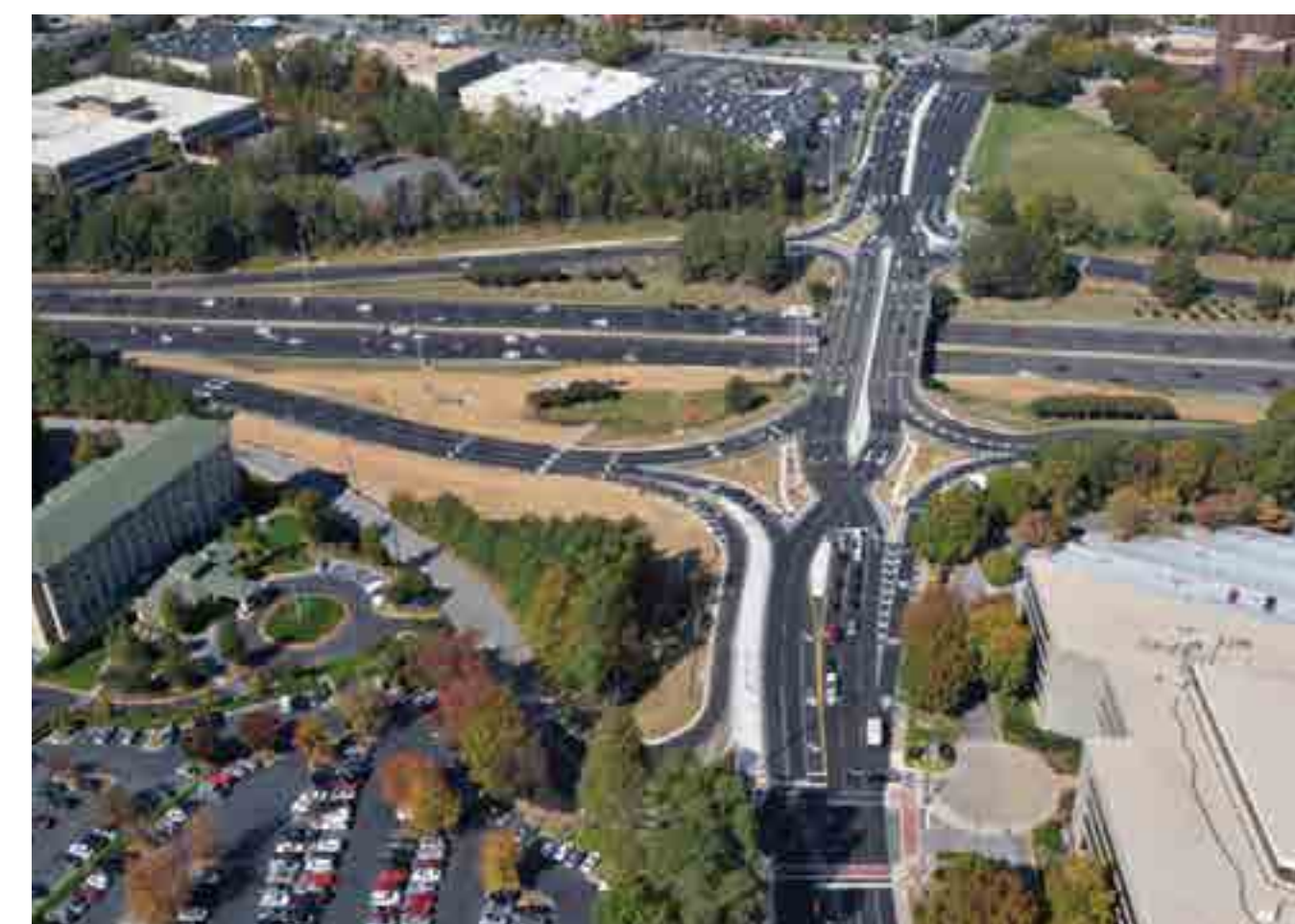
Example: I-285/Ashford Dunwoody Interchange Source: America's Transportation Awards
