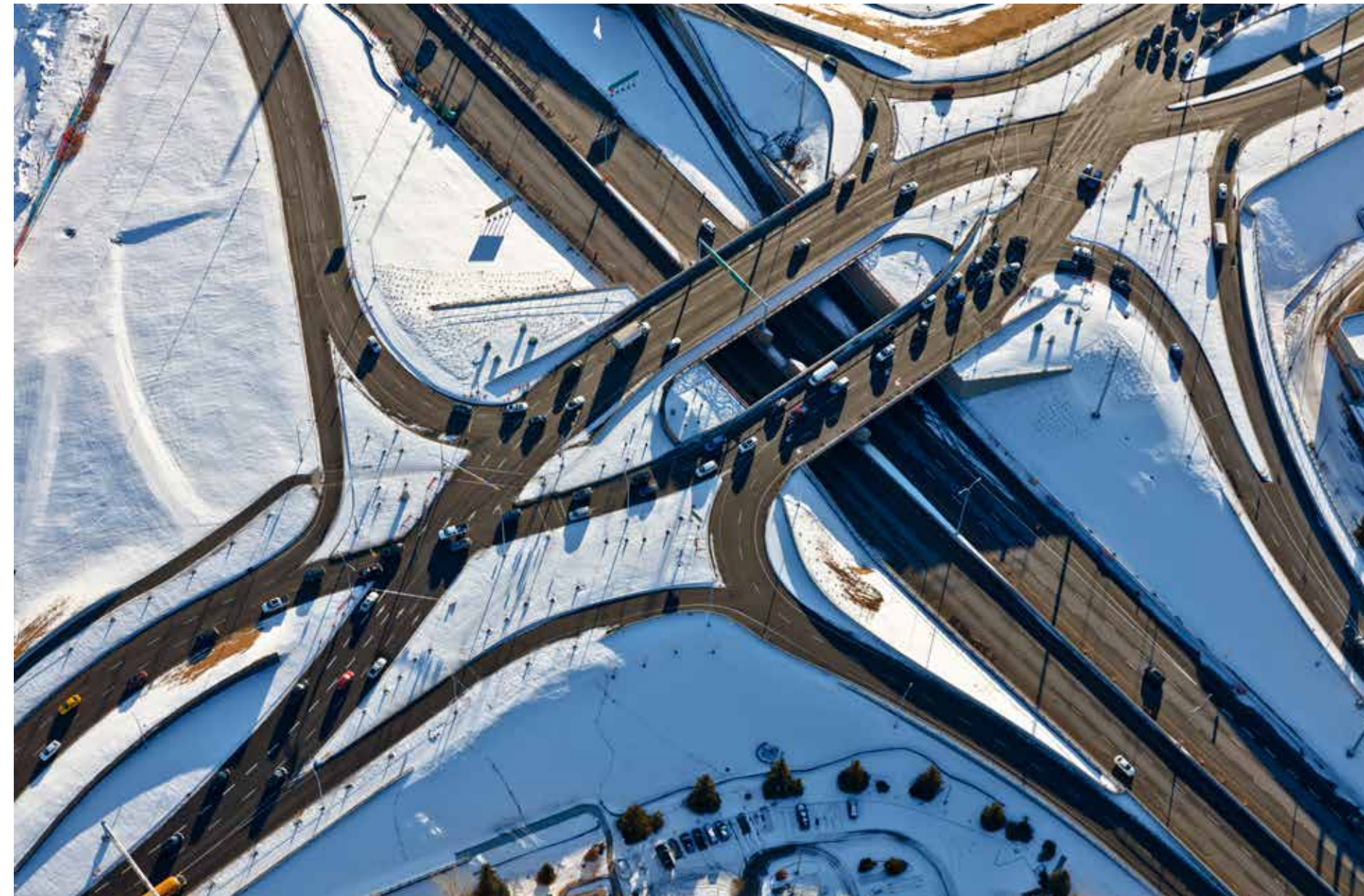
Macleod Tr./162 Avenue S.W. Source: ISL Engineering
