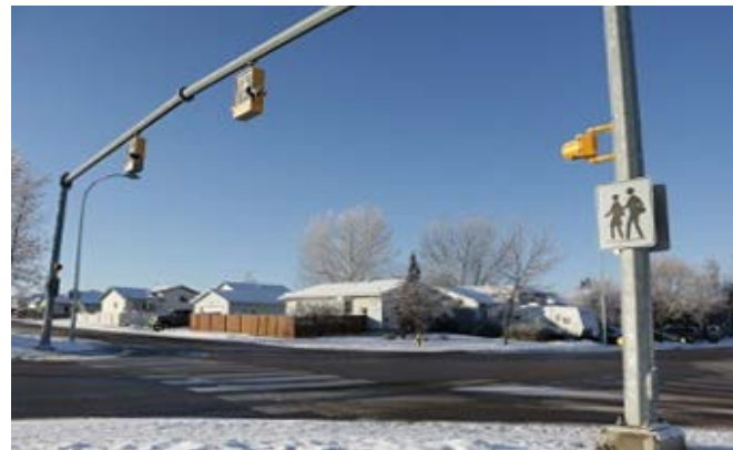
Overhead Pedestrian Flashing Lights
