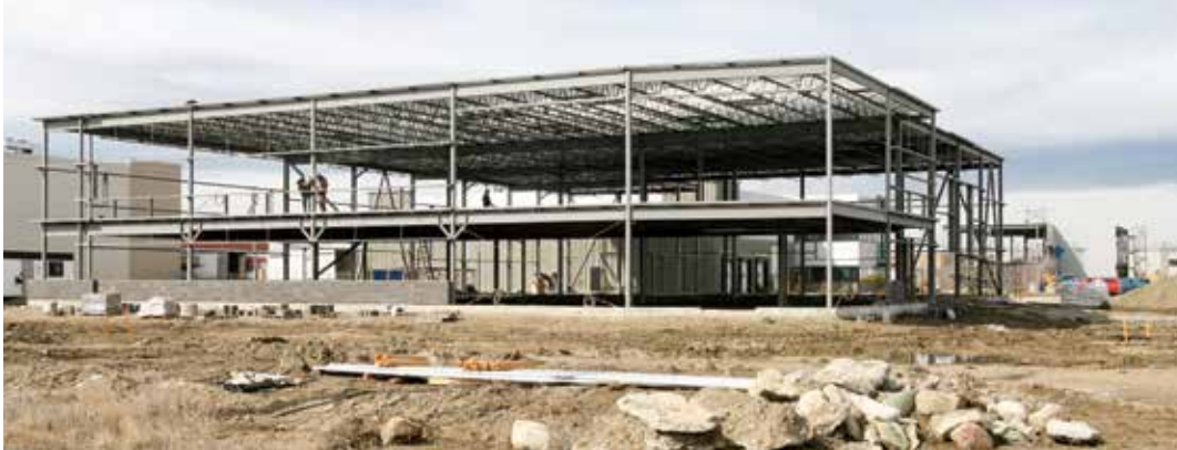
New warehouse under construction in Calgary.
