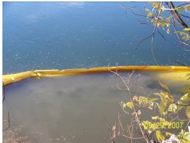
Figure N.3: Turbidity Curtain, Outfall 56, Edmonton Alberta. 2
