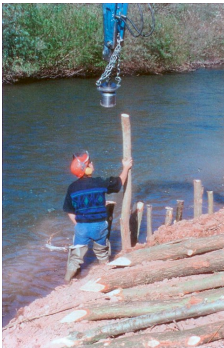
Figure A.1: Fascine with Double Poles – Before and After Installation 1
