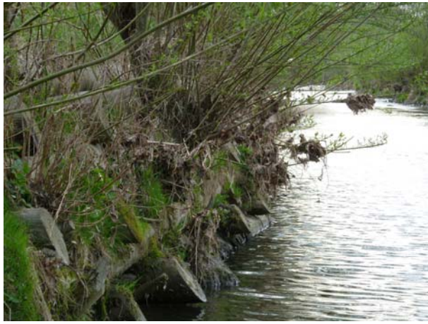
Vegetated crib wall using fascines bundles placed on face of structures. 7
