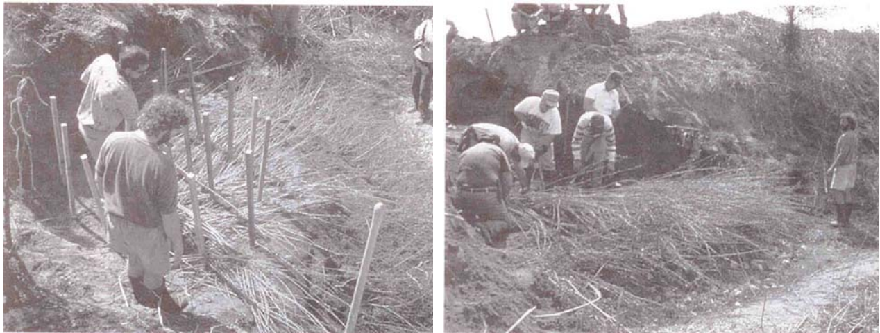
Figure I.13: Branch Packing Installation during Construction 1
