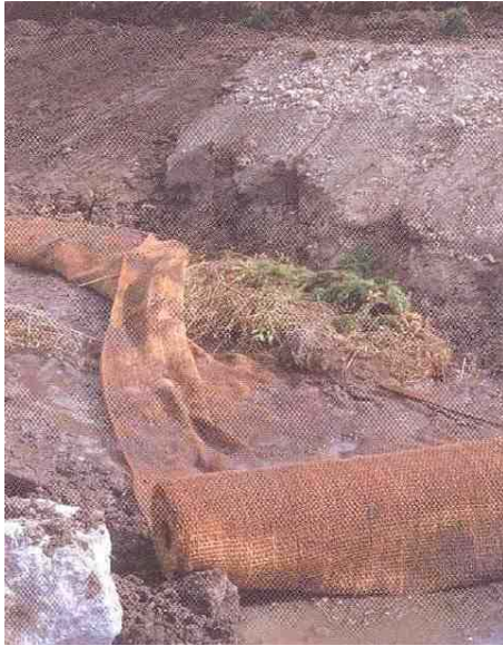
Figure A.4: Aquatic Species Rolls Constructed of Coir Mesh 6
