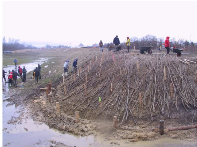
Brush Mattress During Construction
