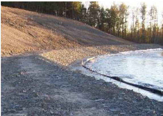
Figure J.5: Heavy Duty Silt Fence Installed in Shallow Water, Salmon River, New Brunswick 5
