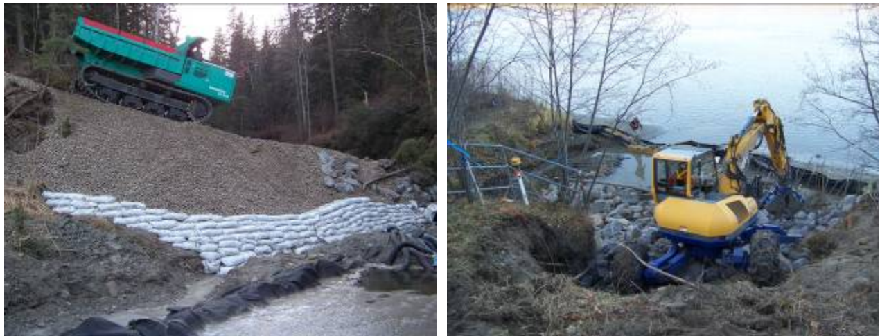
Figure N.2: Tracked Dump Truck and Walking Excavator Working within Riparian/Instream Areas using Biodegradable Hydraulic Fluid. Outfalls 13 & 101, Edmonton Alberta 2
