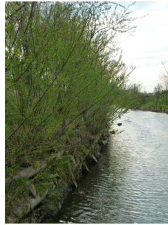
Vegetated crib wall using fascines bundles placed on face of structures. 7
