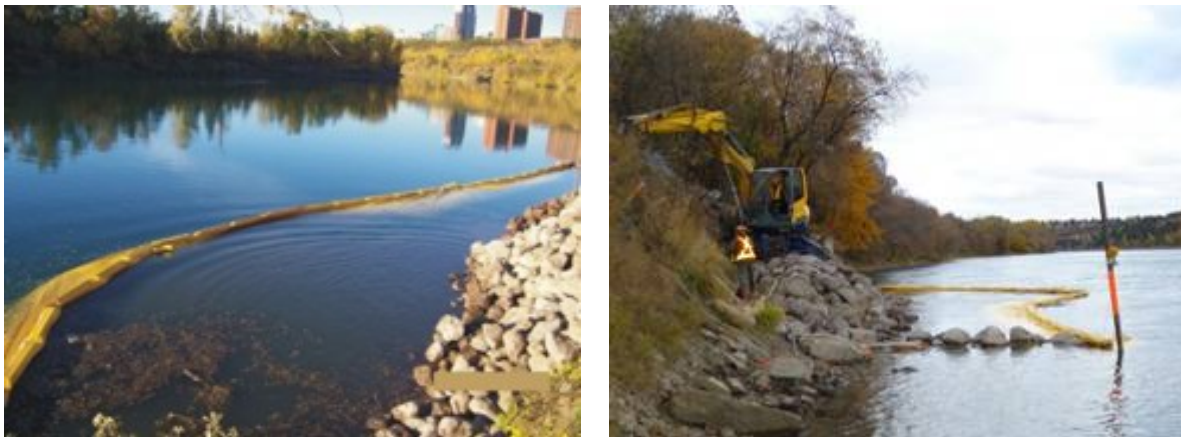
Figure J.6: Floating Turbidity Curtain, Outfall 56, City of Edmonton 6
