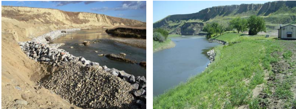
Figure B.1: LPSTP – Construction and After Installation 1
