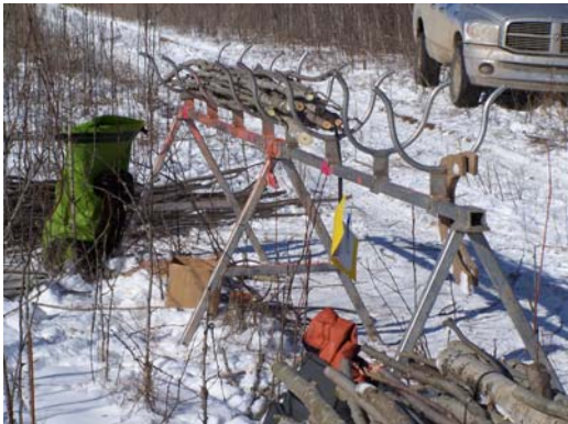
Figure K.1: Bench for Fascine Construction
