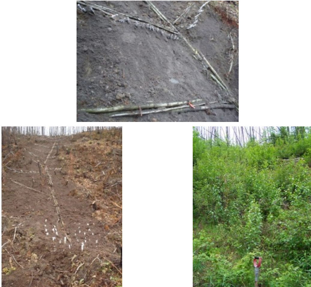
Figure G.1: Installed Live Pole Drains and Same Site with Two Years of Growth 1
