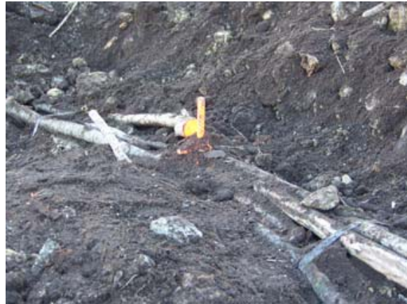
Backfilled Live Fascine 3
