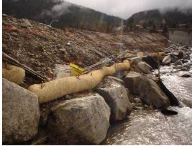
Figure I.9: 12" Straw Wattles Used as Sediment Delivery Prevention along Rocky Shoreline 2
