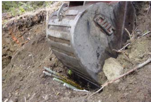
Figure I.1: Brush Layer Installation 1
