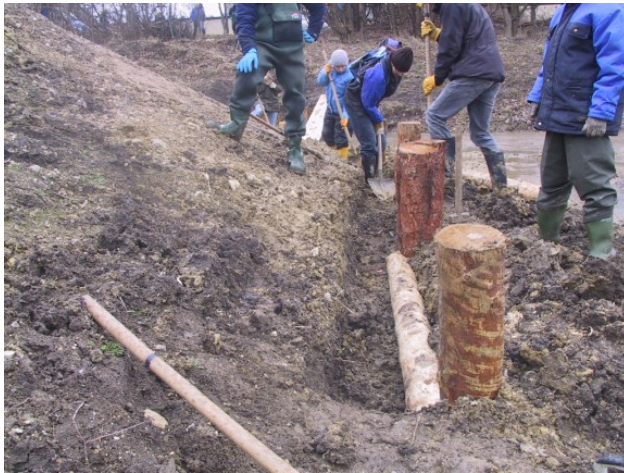
Brush Mattress Log Toe Construction
