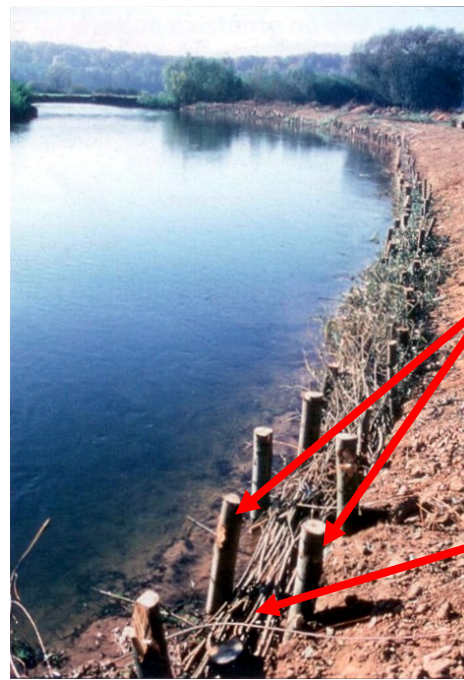
Figure A.1: Fascine with Double Poles – Before and After Installation 1
