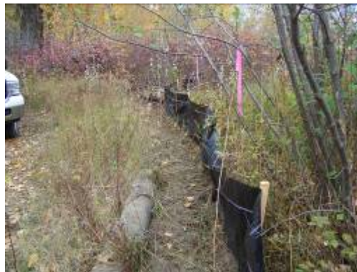
Figure J.9: Installed Silt Fence 12
