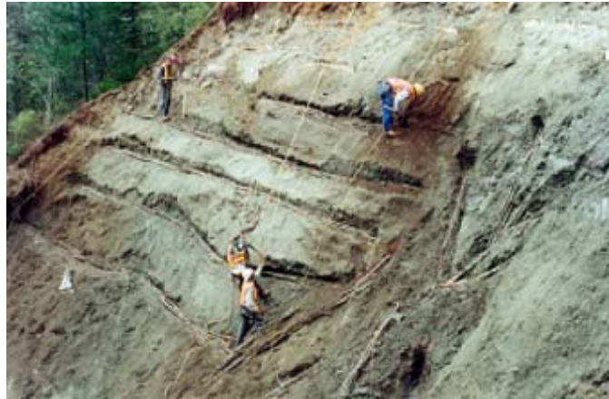
Installation of Fascines Rows on Steep Slope 1
