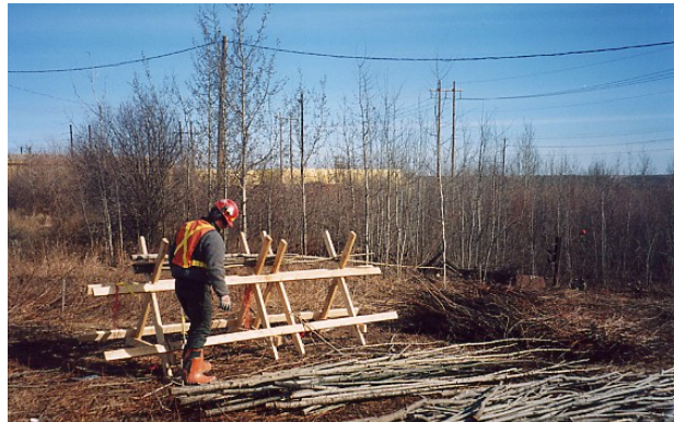
Figure K.1: Bench for Fascine Construction
