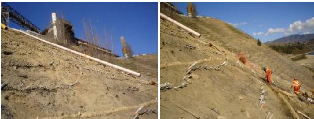
Figure I.12: Transport of straw wattles on steep slope with access on top of slope 5
