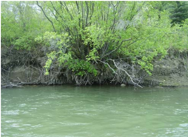
Figure Q.1: Example of Undermined Bank with Excellent Overhanging Native Woody Vegetation 1
