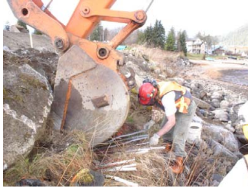
Figure F.3: Planting of existing riprap using excavator bucket 4
