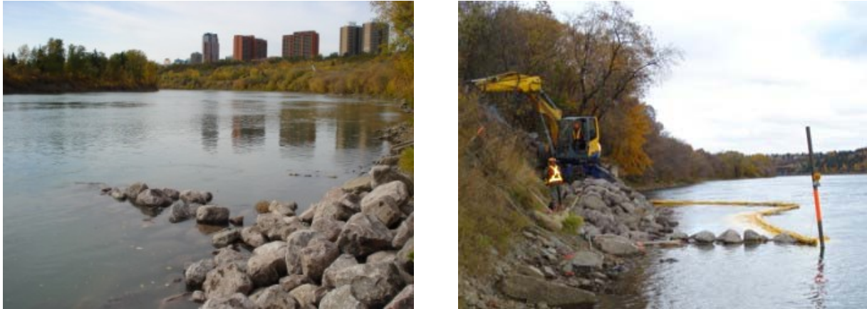
Figure O.2: Constructed Rock Vane and Temporary Rock Vane Used to Anchor Floating Turbidity Curtain 7
