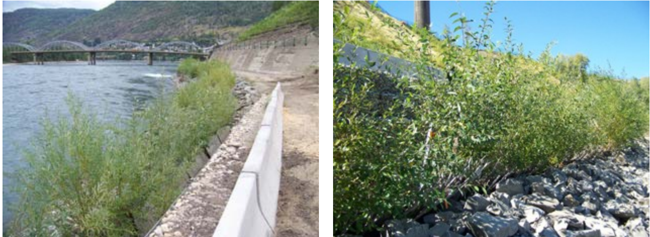
Figure D.1: Vegetated Riprap with Toe Apron and One Vegetated Row 1
