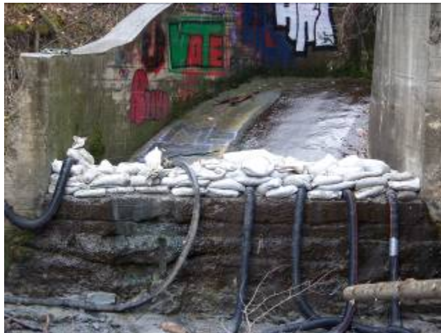
Figure J.2: Sandbag Cofferd Dam, Using Sand Bags and Big-O-Pipes, Willow Creek Ravine, Outfall 13, City of Edmonton 2
