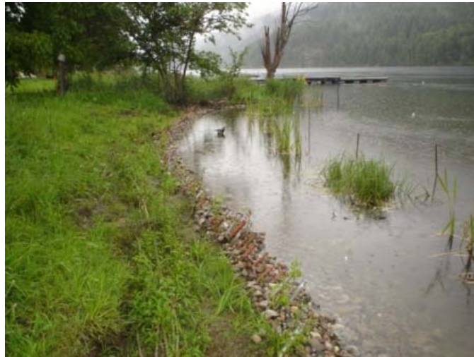
Figure C.1: Rock Toe with One Brush Layer Row, Contour Fascine and Aquatic Species 1
