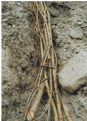
Figure G.3: Fascine Bundle with “T” Rebar 3
