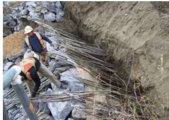
Figure D.3: Installation of Vegetated Row 4
