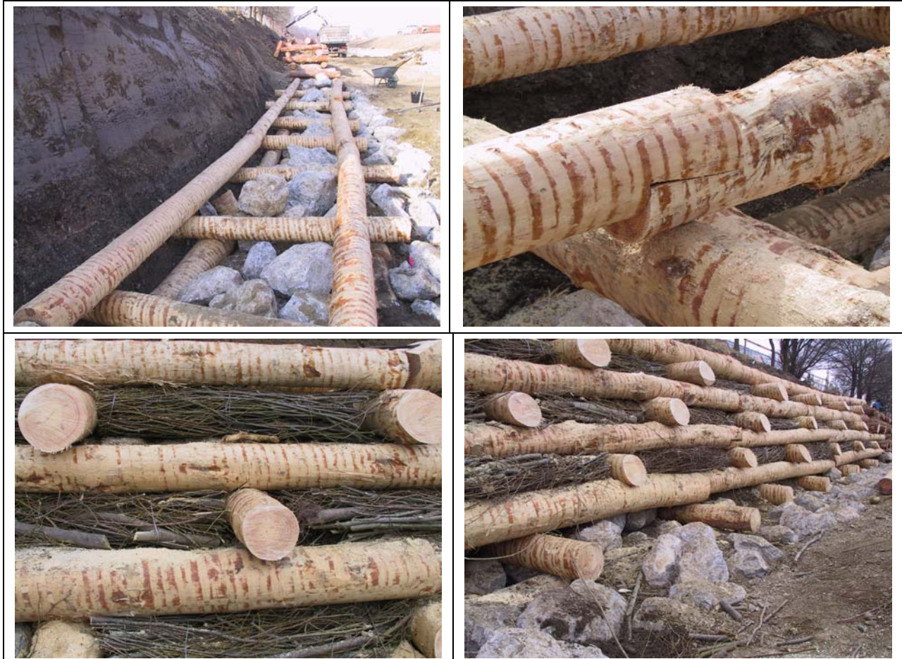
Vegetated crib wall construction using fascines bundles placed on the face of the structures. 6
