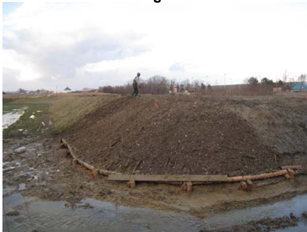
Brush Mattress After Backfilling
