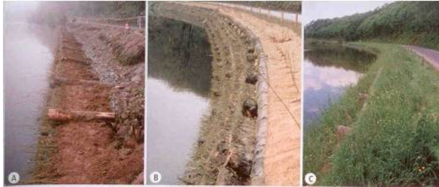
Figure E.1: Overview Vegetation Establishment at Log Crib Wall
