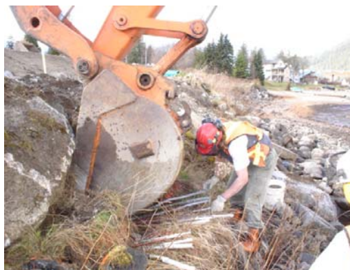
Figure C.3: Machine assisted brush layer planting 3
