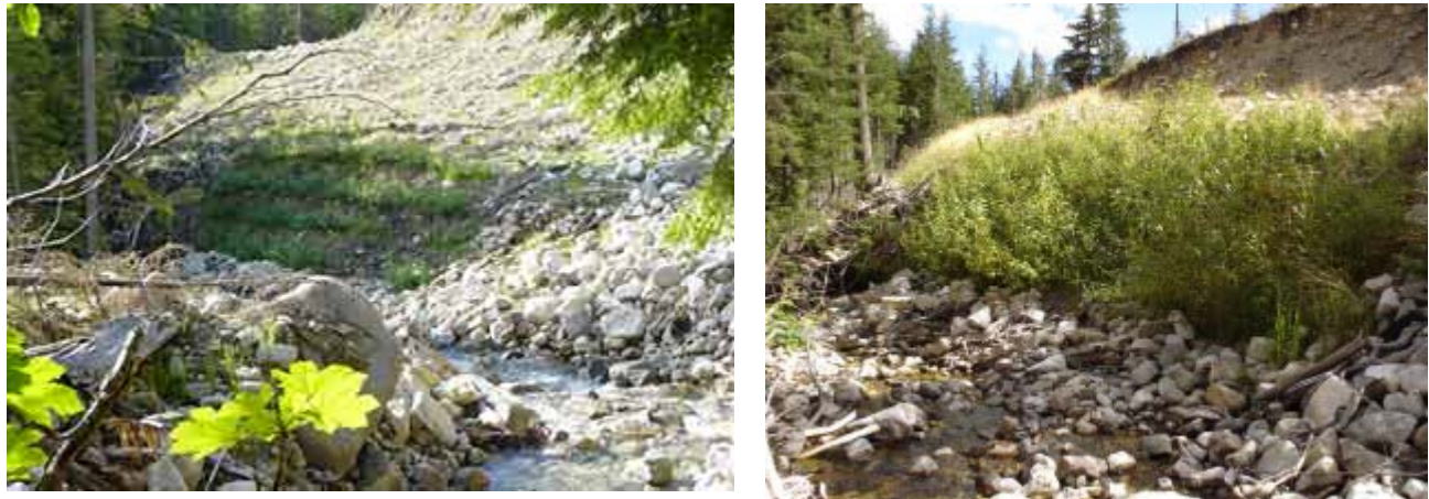
Figure C.5: Rock Toe with Multiple Brush Layer Rows and Contour Fascines 8
