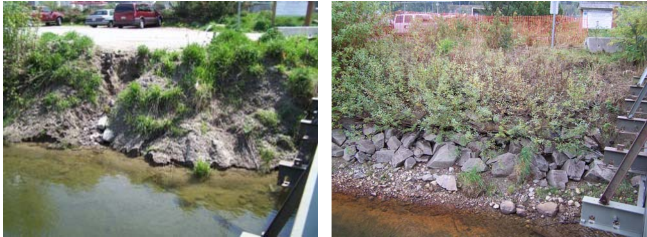
Figure D.4: Vegetated Riprap Before and After 5
