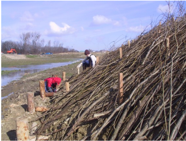
Brush Mattress Installation 1
