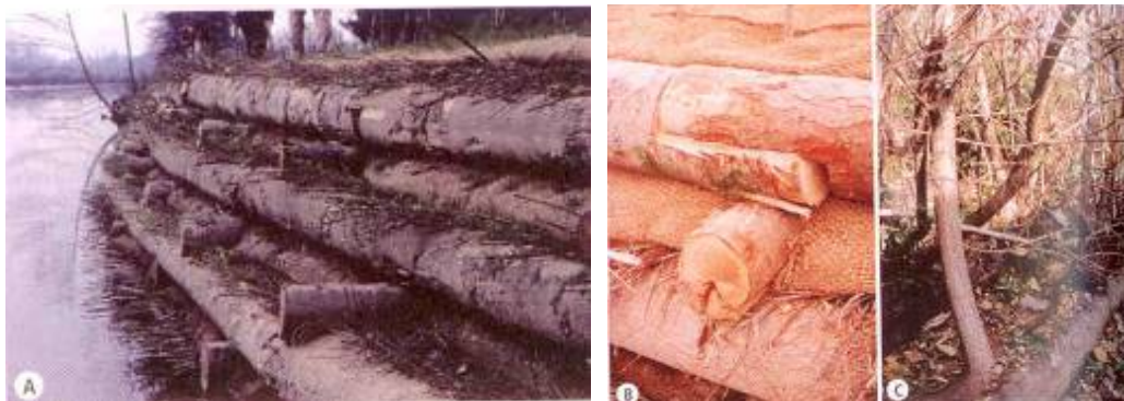
Figure E.2: Detail Vegetation Establishment at Log Crib Wall
