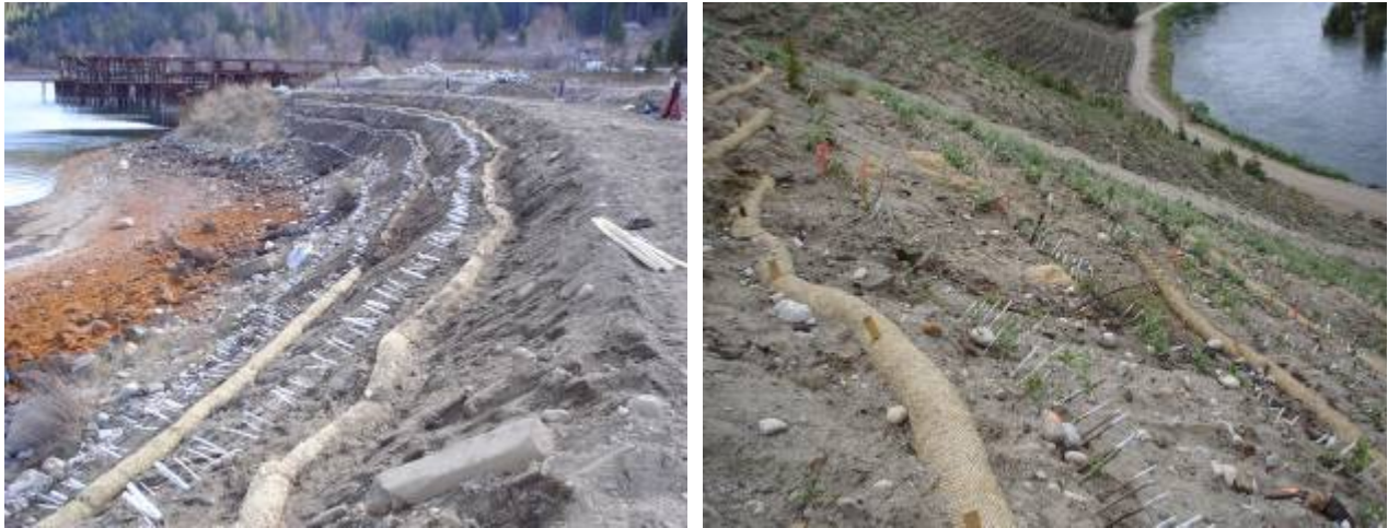
Figure I.8: Installed Straw Wattles, Streambank and Riparian Applications 1
