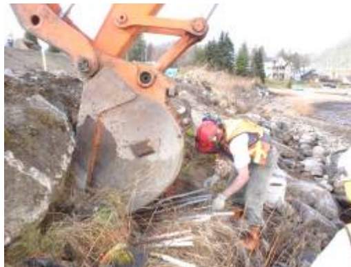
Figure I.4: Machine assisted brush layer planting 5
