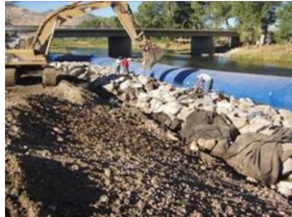
Figure J.4: Water Inflated Dam 4
