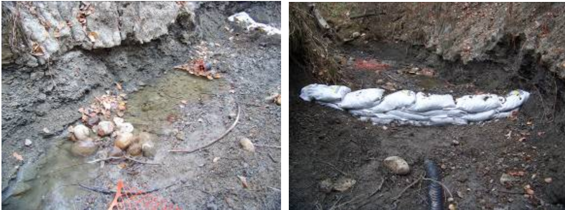
Figure J.1: Earth / Sandbag Cofferd Dam, Intake and Outlet Willow Creek Ravine Outfall 13, City of Edmonton 1
