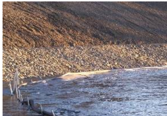
Figure J.5: Heavy Duty Silt Fence Installed in Shallow Water, Salmon River, New Brunswick 5
