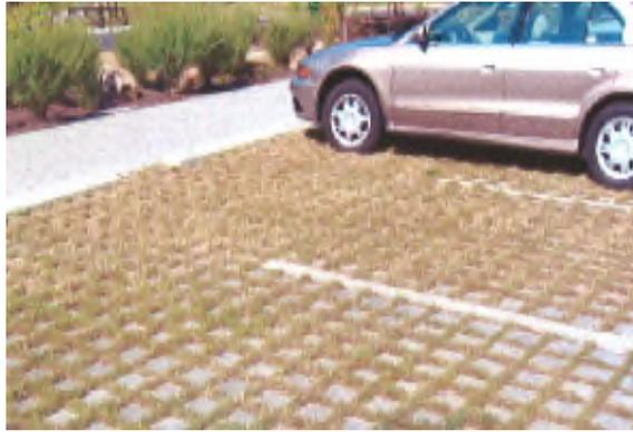
**Figure 10: Concrete Grid Porous Pavers**
