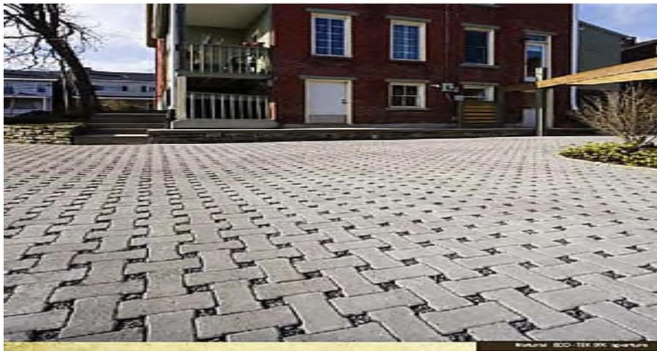
Figure 7: Interlocking Shapes with Openings
