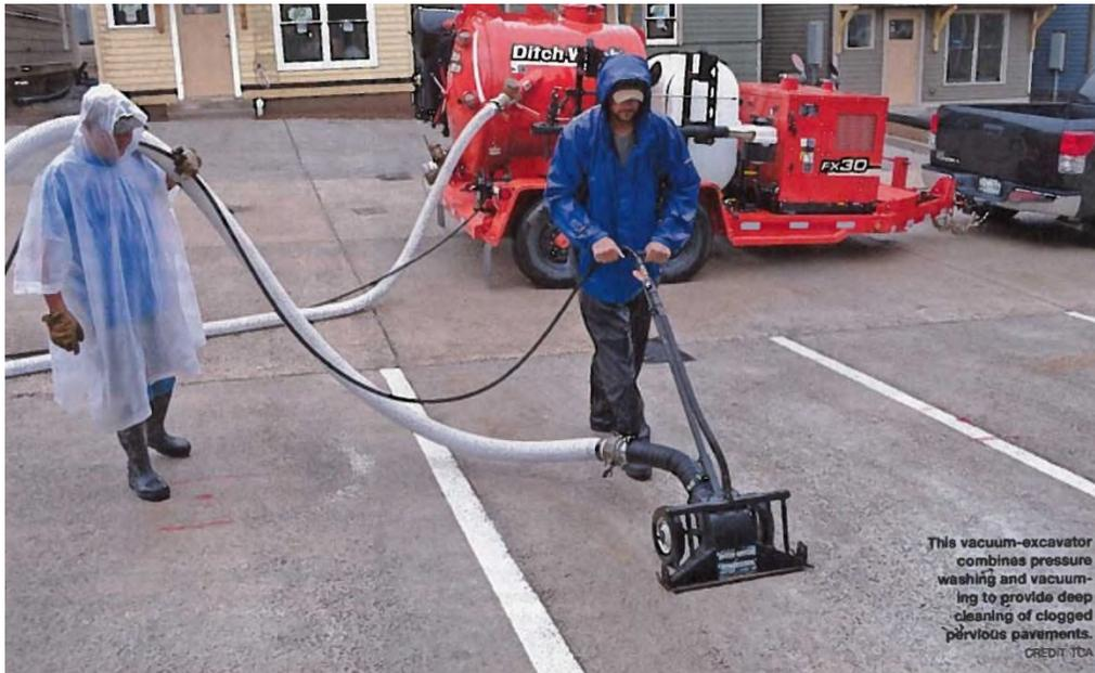
Figure 12: Pressure Vacuum and Washing Equipment (Courtesy of Concrete Construction June 2013)
