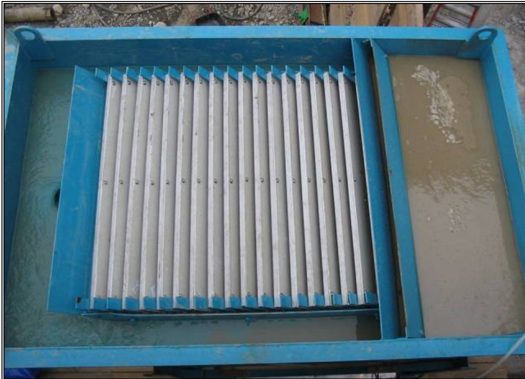
Photo 18: Inclined Plate Clarifier Tank commonly used for construction dewatering sediment removal in Calgary. The tank inlet is on the right and the outlet on the left.
