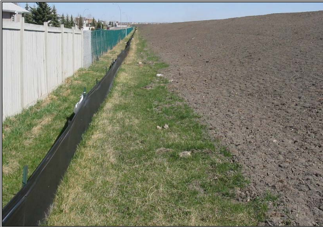
Photo 8: Use of a vegetated buffer strip in combination with a perimeter silt fence and a topsoiled and tracked slope. BMPs work most effectively if they are implemented as part of a system of erosion & sediment control.
