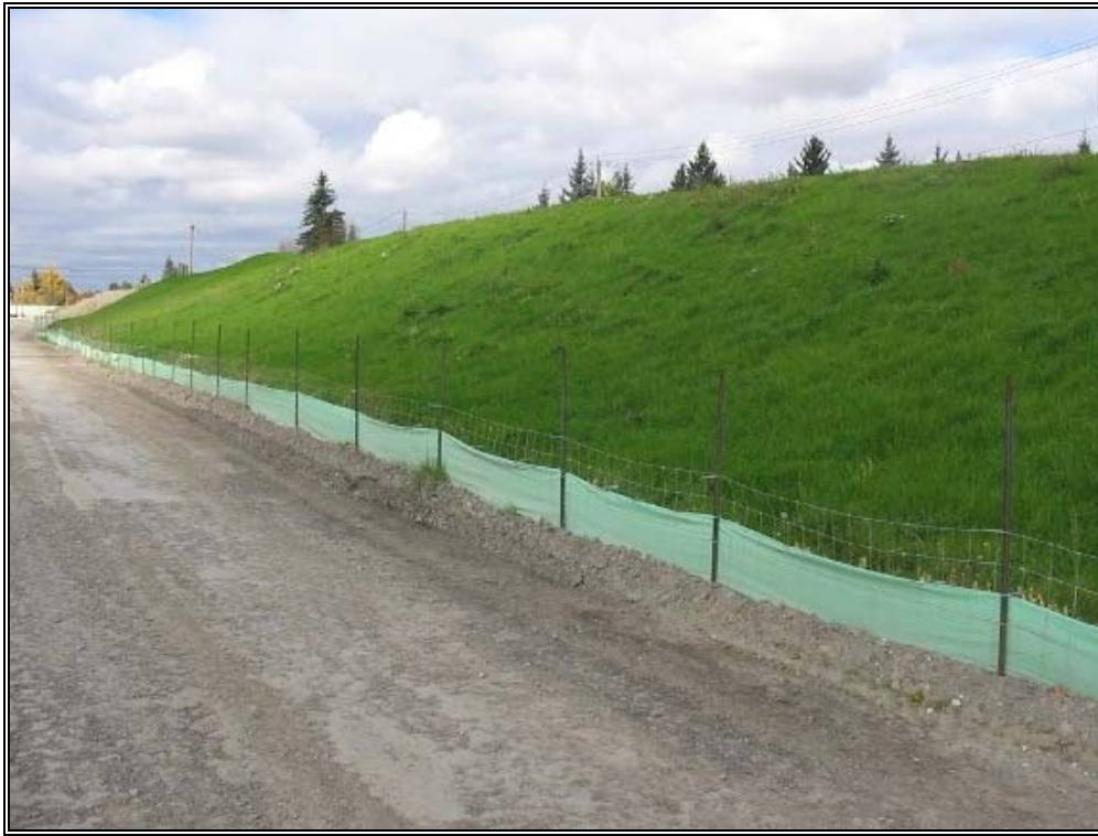
Photo 9: Providing vegetation cover on this soil stockpile controls erosion and helps preserve the biological, chemical and physical integrity of the soil. Perimeter control (silt fence) was installed around the pile to control migration of sediment during stabilization.
