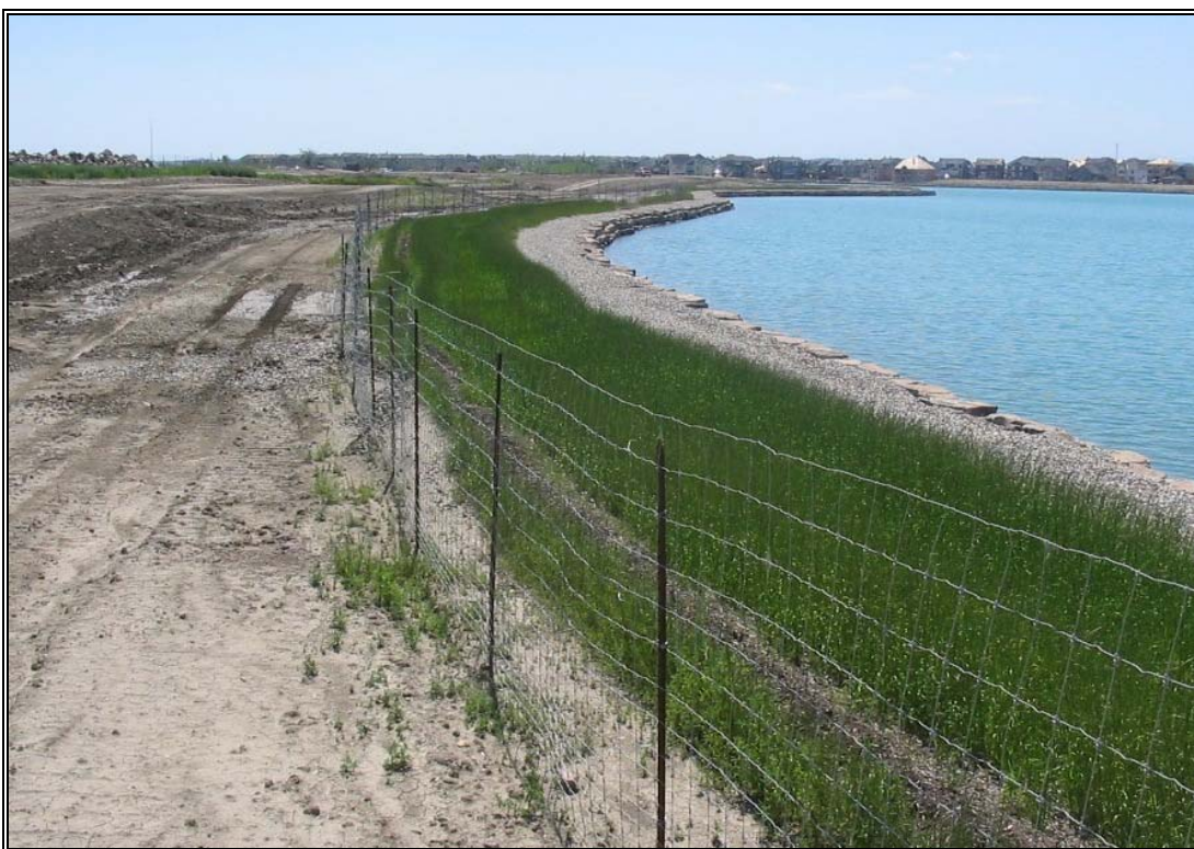
Photo 13: Protection of water body adjacent to a stripped area of land is enhanced with a seeded compost berm and compost blanket (promotes filtering of sediment-laden run-off and provides an erosion-resistant buffer.
