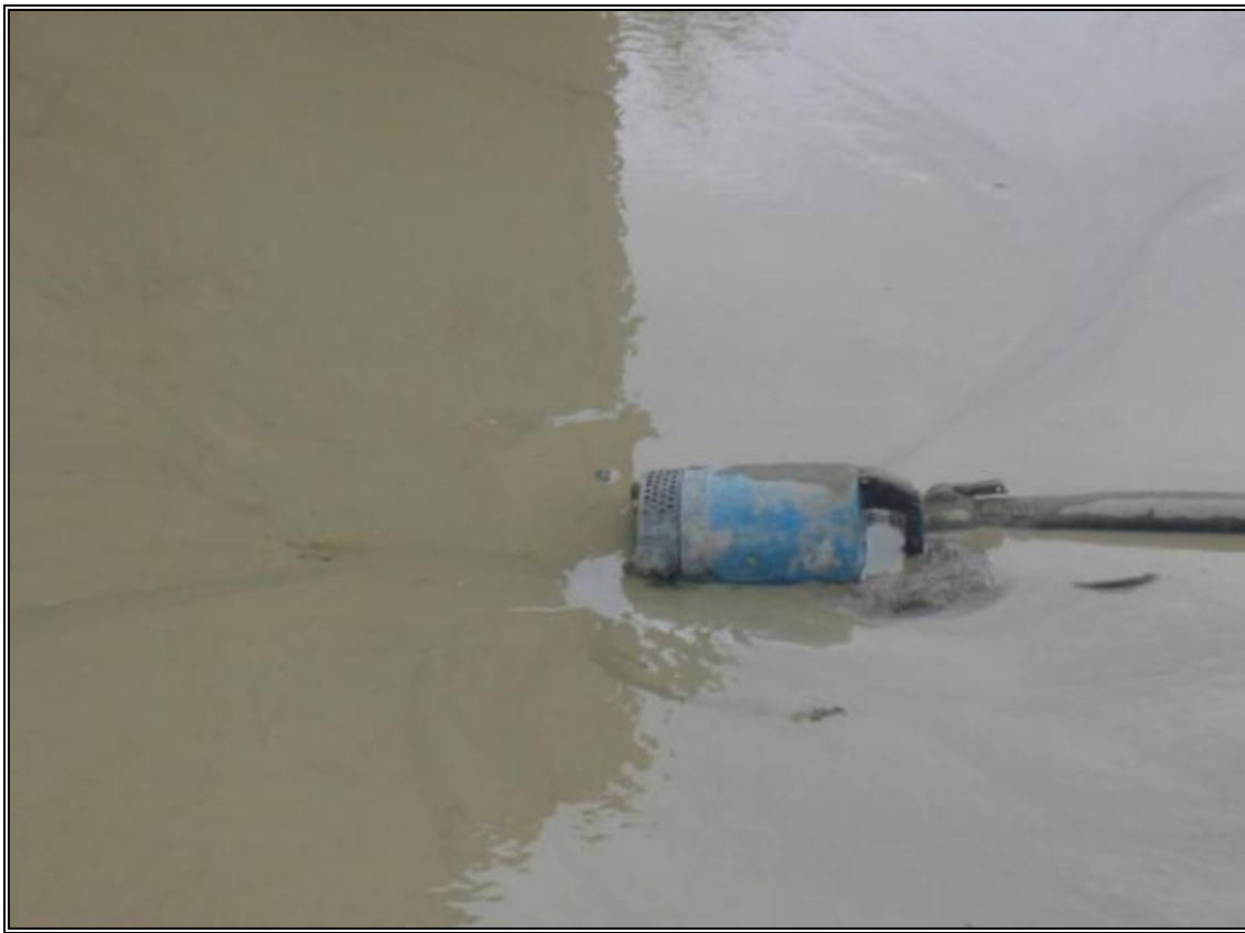
Photo 17: Uncontrolled dewatering of this sediment trap to a storm sewer resulted in a sediment release and the cancellation of the drainage permit for the construction site.
