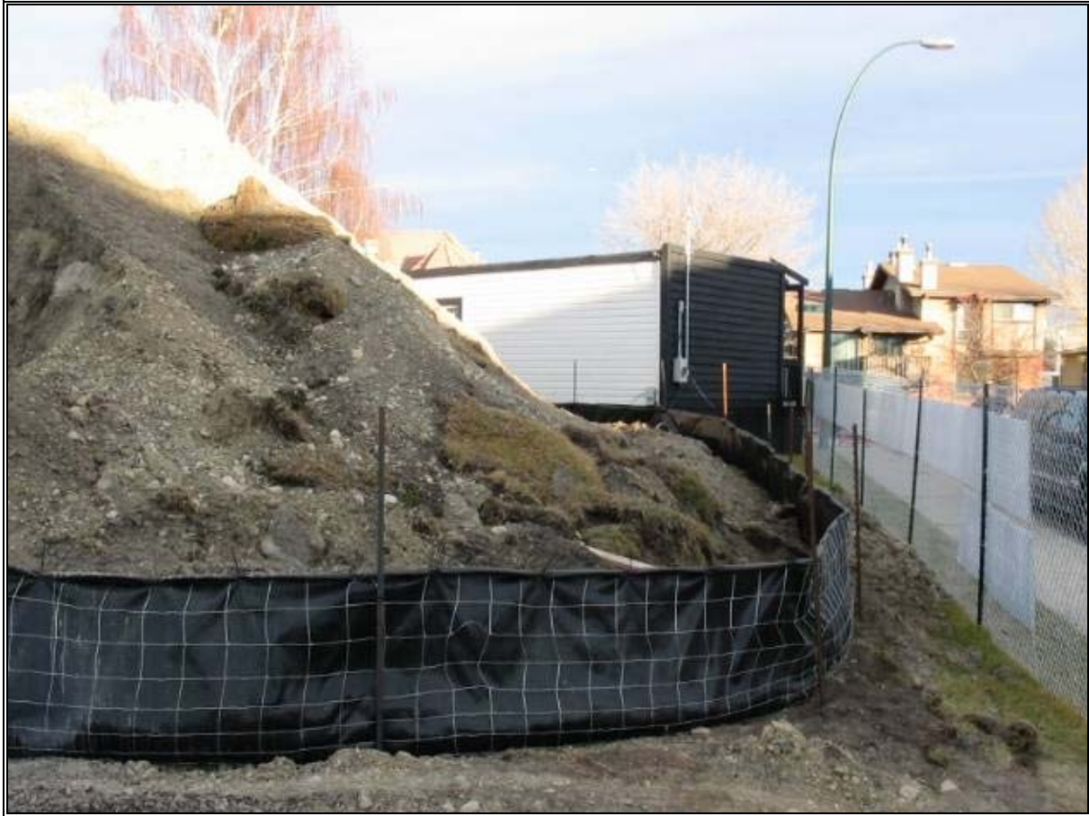
Photo 5: Placement of silt fence around a temporary stockpile on a multi-family development. Note that long term stockpiles such as this one should also be stabilized with vegetation or other temporary cover.
