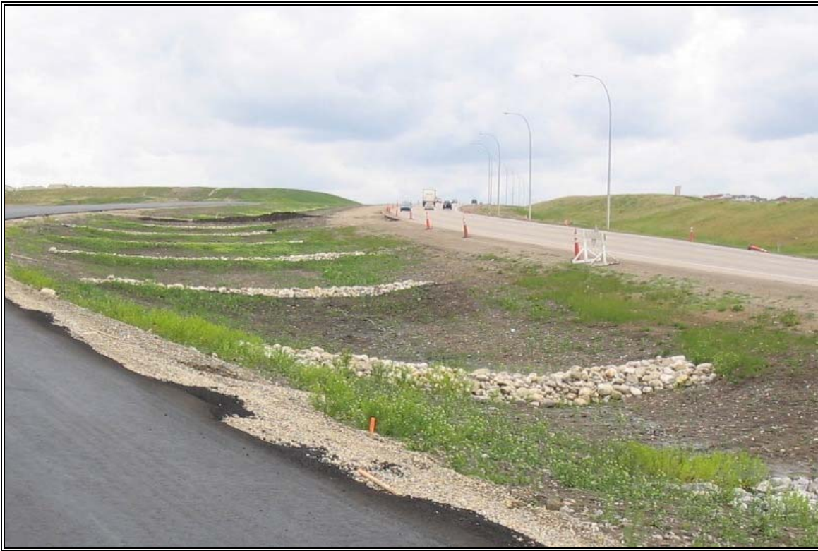
Photo 11: A system of well-installed rock check dams (properly spaced and extended up the sides of the channel) on a road construction project.
