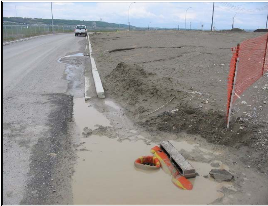
Photo 22: Storm inlet protection, such as the device shown in this picture, will fail if source controls (erosion, run-on and run-off controls) are not properly planned or implemented. There are no source controls implemented on the construction site shown in this photo.
