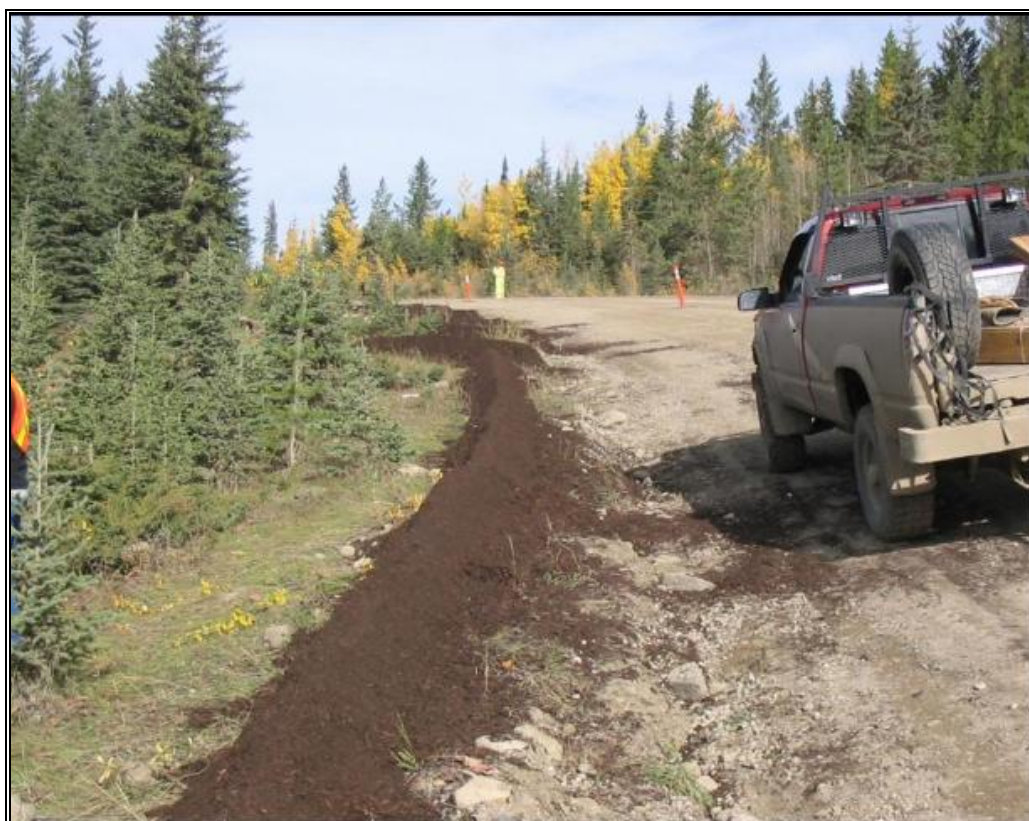
Photo 14: Installation of a compost berm
