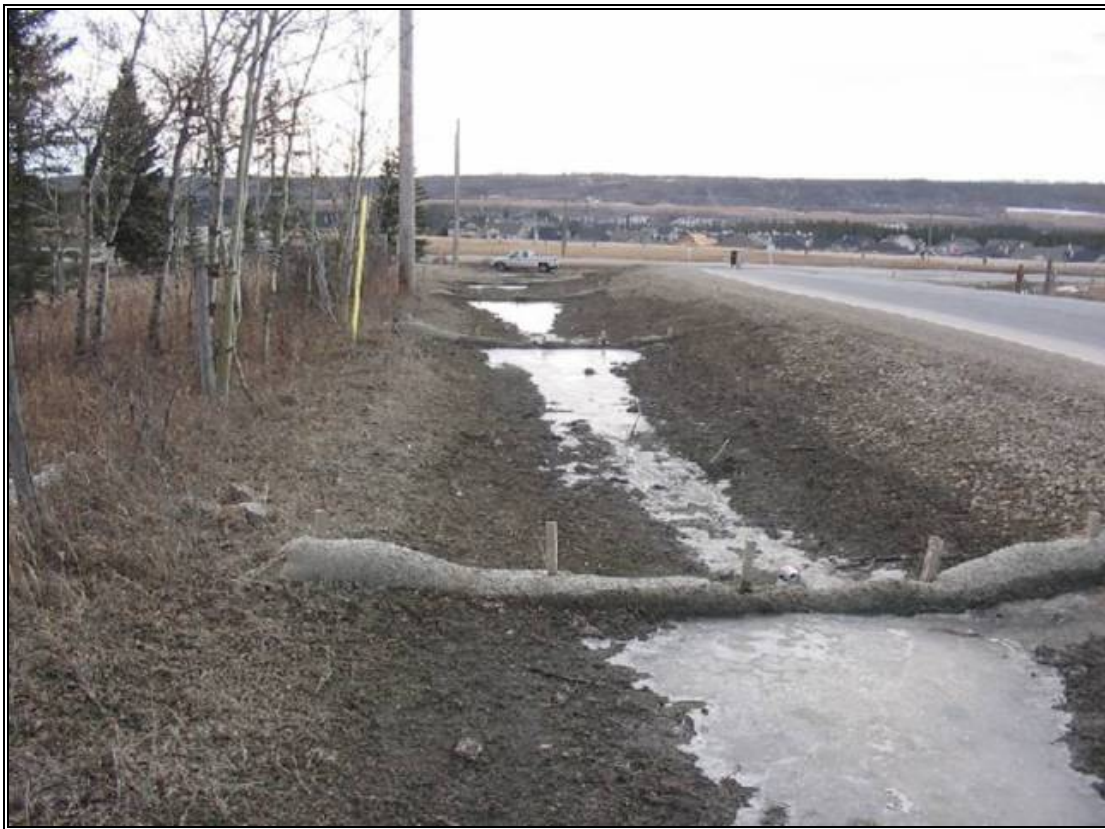
Photo 15: Straw wattles provide an excellent type of ditch check in small ditches conveying small volumes of run-off.
