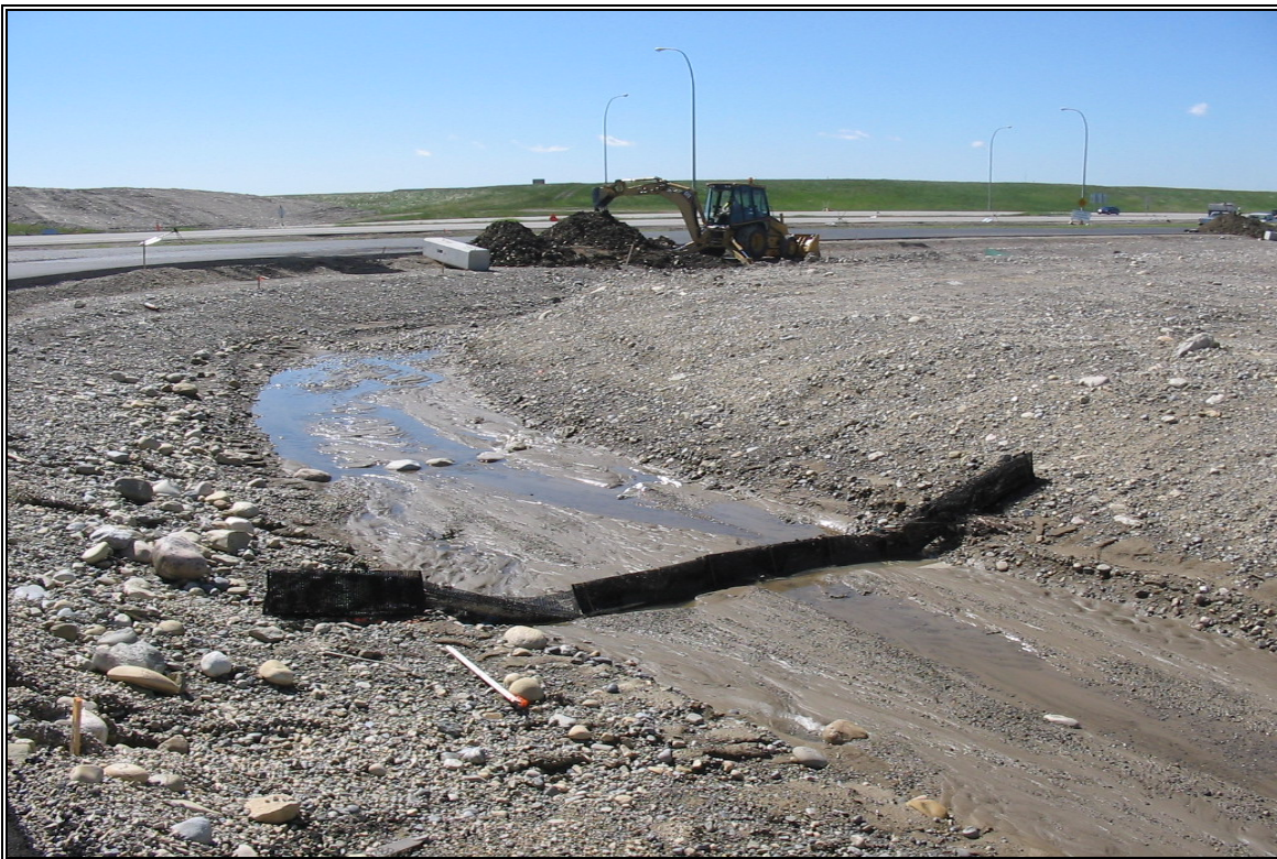
Photo 12: Ditch checks can be subject to washout and undermining if not properly installed (spacing, anchoring, and configuration) or used as part of a system of erosion & sediment controls.
