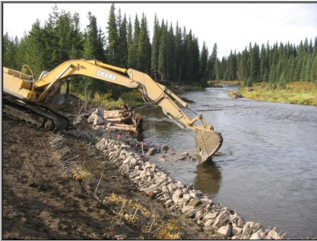
Photo 16: Streambank Biotechnical/Bioengineering Project on the Pembina River, west central Alberta (note the use of brush layering, riprap toe protection and rock vanes).
