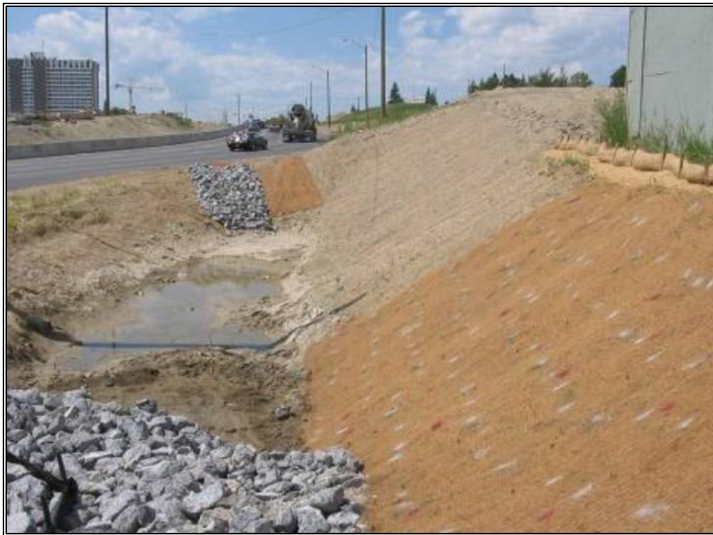
Photo 20: Simple sediment trap, with stabilized inlet and outlet and application of an erosion control blanket to protect side slopes.
