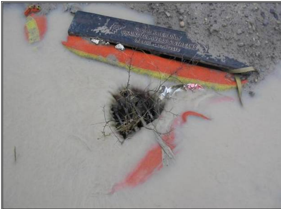
Photo 23: Release of sediment-laden water from a construction site into a storm sewer during a minor rainfall event. In addition to potential enforcement by provincial and federal regulators, the specified penalty under The City of Calgary Drainage Bylaw 37M2005 for causing a release of a Prohibited Substance (sediment) is $3,000 per offence (each day constitutes a separate offence). Court imposed fines can go up to $10,000 per offence.
