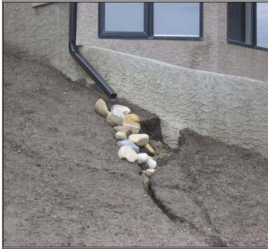
Photo 3: Discharge from downspouts is a common cause of erosion of unstabilized soils. In this case, rock has been added in an attempt to control erosion. All downspouts are required to discharge to a suitably sized stabilized area such as vegetation or a properly installed energy dissipater (riprap or other material).
