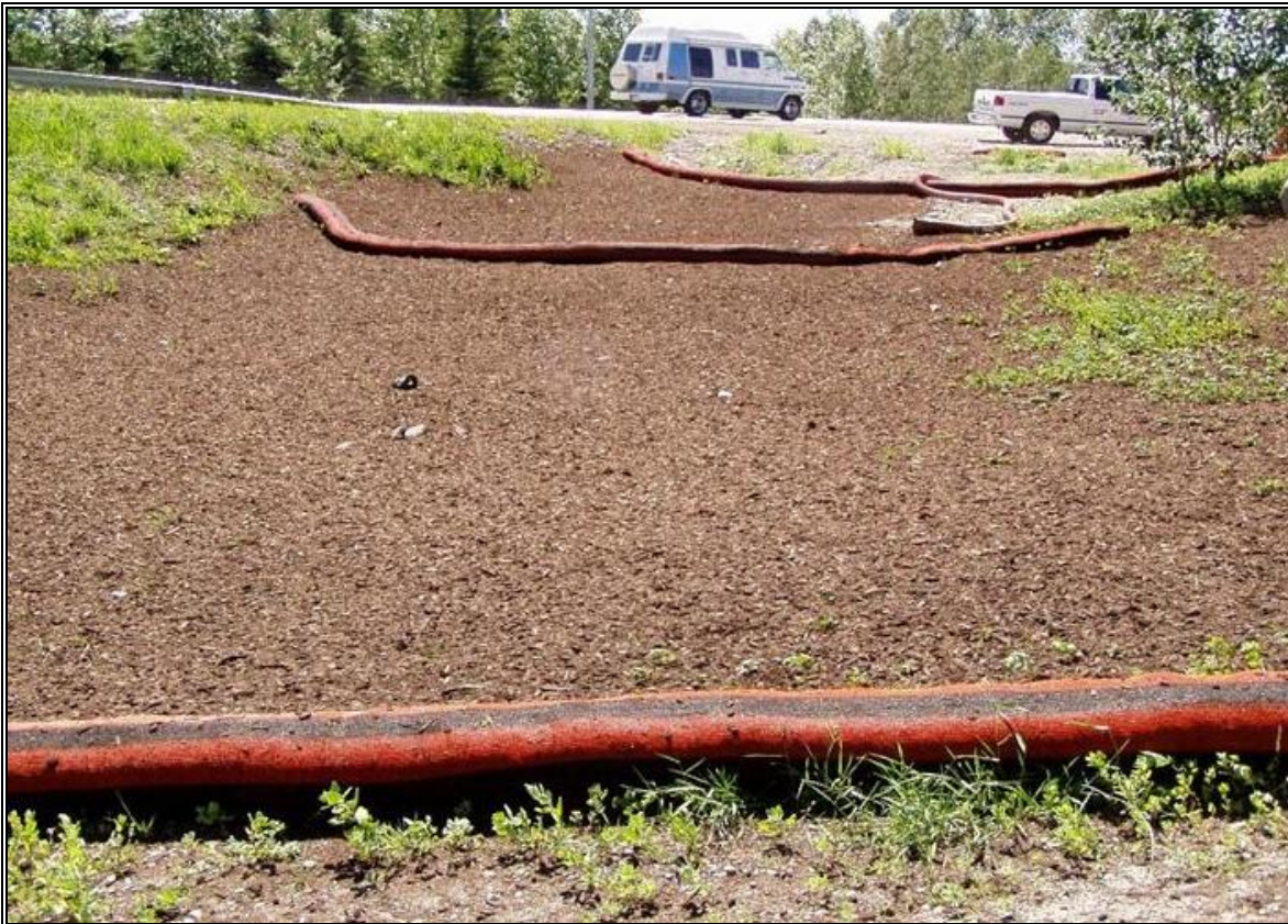
Photo 21: Combination of compost socks and a compost blanket applied to control erosion adjacent to a sensitive creek. A design seed mix was incorporated with the application, resulting in long-term erosion control. Biodegradable compost sock liners are also available.
