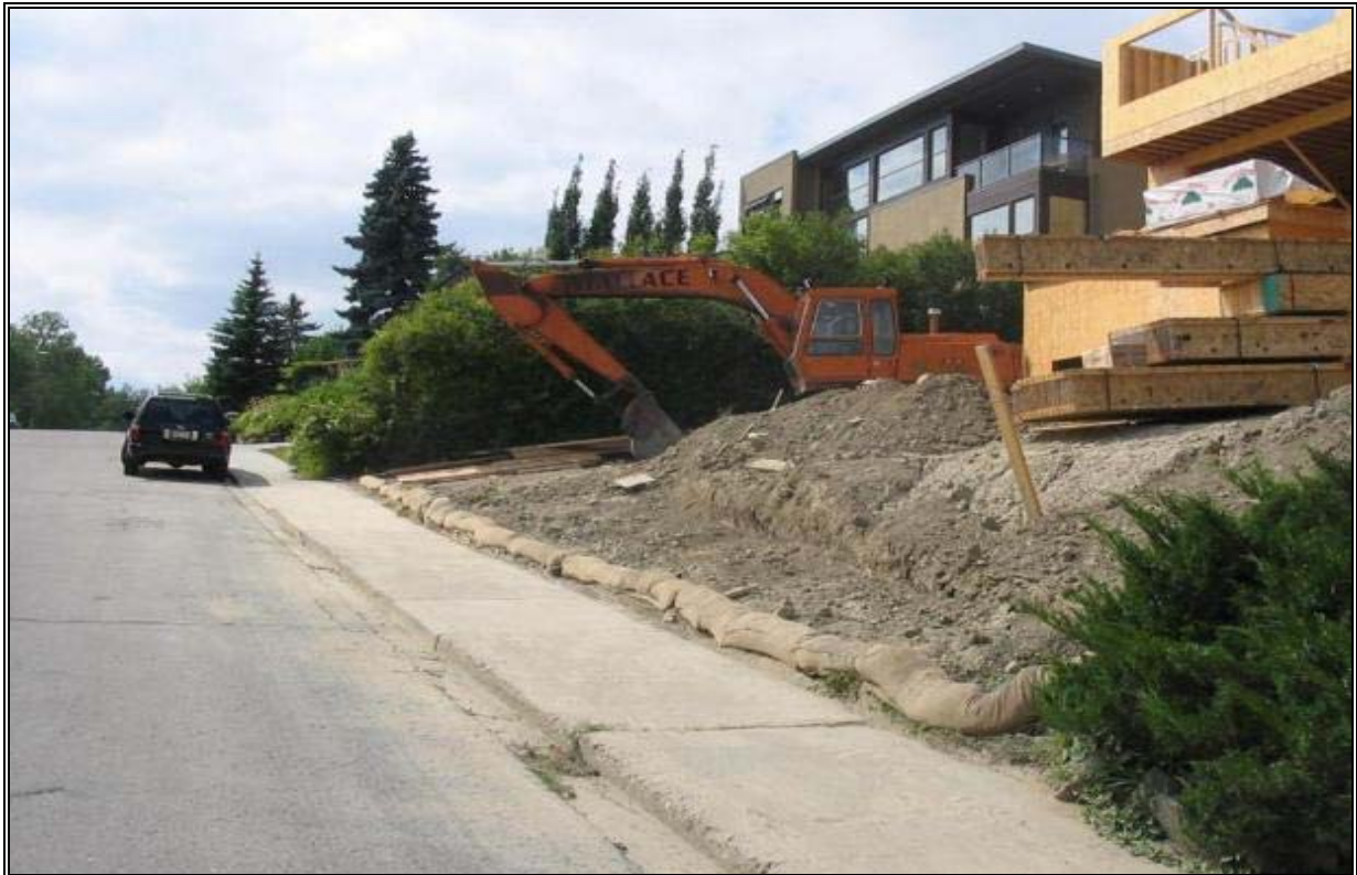
Photo 7: Placement of wood chip filled bags as a lot log perimeter control on a steeply graded lot. Note that a temporary v-ditch sediment trap must be excavated on the upstream side of the lot log and the bags better entrenched and staked into place to prevent sediment-laden flow undermining this control.
