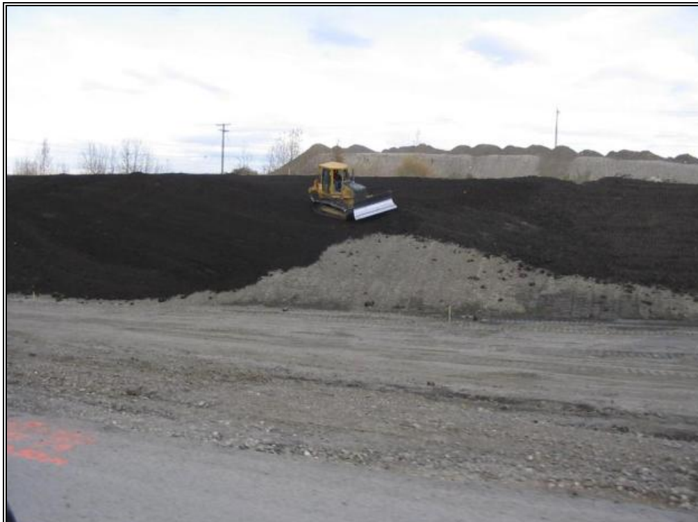
Photo 10: Timely final grading and site preparation, followed by application of topsoil reduces the exposure of highly erodible subsoil to erosion. Upon completion of topsoil application, additional erosion control measures detailed in the Erosion & Sediment Control Plan should be implemented.
