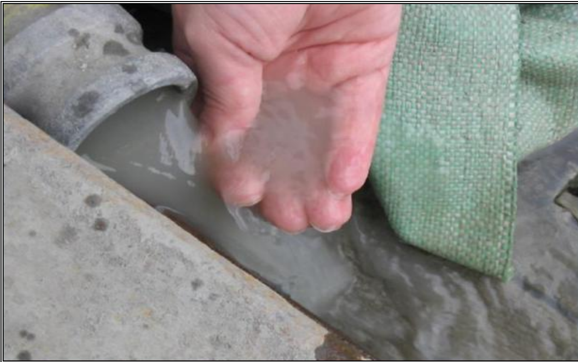
Photo 19: Monitoring discharge turbidity during construction dewatering or drainage is critical. The discharge in the photo is in downtown Calgary and is entering a storm sewer catchbasin that drains to the Elbow River. Given river background levels of 3 to 4 turbidity units (NTU), this water (345 NTU) is too turbid to be discharged to storm. Typical Drainage/Dewatering Permit conditions require that a dewatering discharge to a catchbasin should never exceed 50 NTU.
