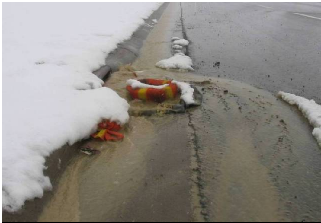
Photo 24: This storm inlet sediment control device has been installed on a grade, resulting in downstream diversion of sediment-laden run-off during a snow melt event. Construction site soils left exposed over winter must be stabilized and run-off from construction sites controlled at all times. Storm inlet sediment controls must not be placed such that they could cause downstream diversion, flooding or other hazardous conditions.
