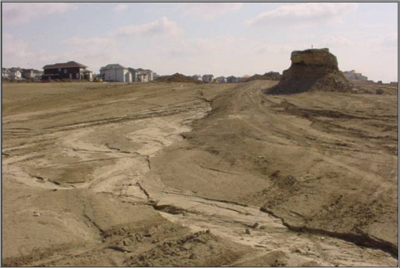
Photo 1: Without practices in place to control run-on/run-off, stabilize soils and capture eroded sediment, excessive removal of vegetation and topsoil can lead to compaction and erosion of fine-grained soils, exponential increases in surface run-off and off-site discharge of sediment-laden water and dust.
