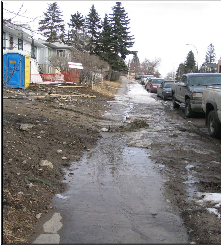
Photo 4: Uncontrolled run-off and erosion from inner city infill development resulting in off-site sediment releases and sedimentation.
