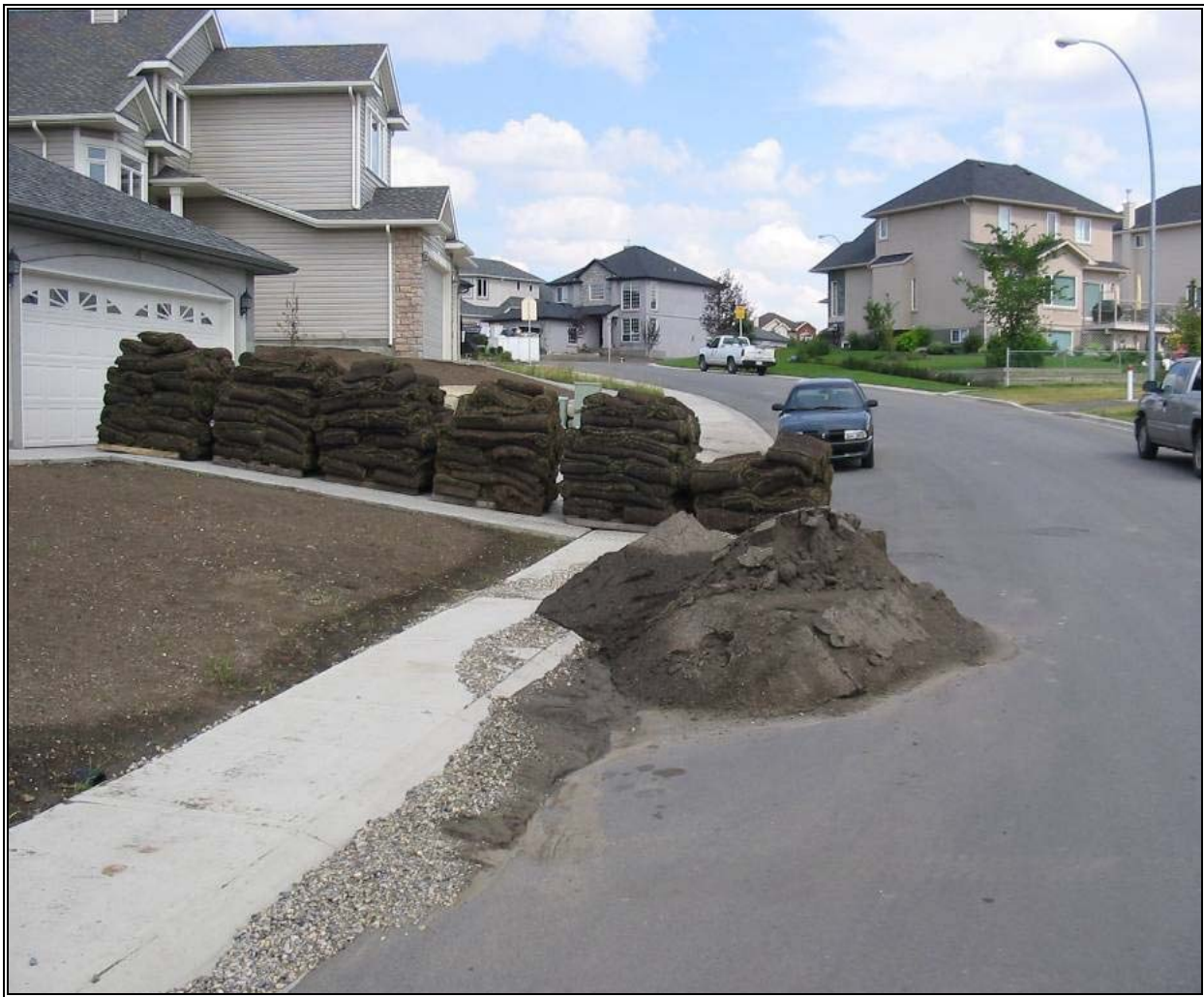
Photo 6: Uncontrolled stockpiling on a street, causing erosion of pile material and a resulting release to the storm sewer. Note that The City of Calgary Drainage Bylaw 37M2005 provides for a specified penalty of $3,000.00 for releasing prohibited substances such as sediment to a storm sewer.
