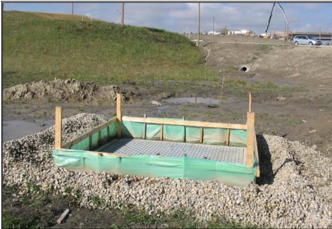
Photo 25: Rock weepers can increase the effectiveness of other temporary inlet sediment controls.
