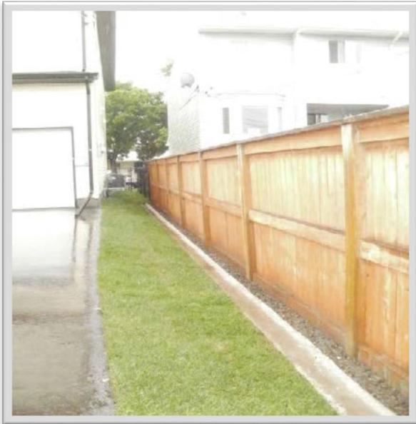
Figure 24 – Concrete Swale at Side Yard. Source: The City of Edmonton Lot Grading Guidelines
