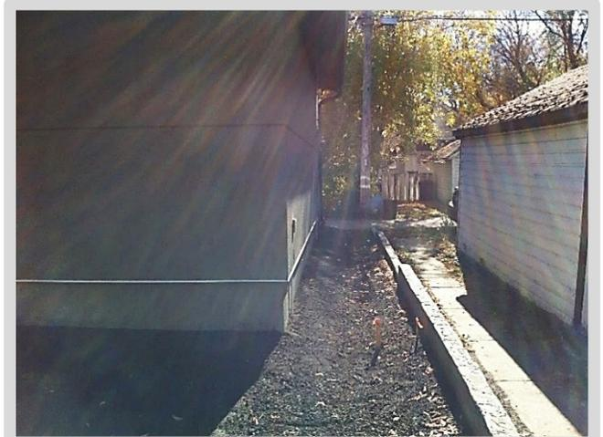
*Figure 14 – Infill redevelopment with higher lot elevations than adjacent property manages lot drainage with Swale and Retaining Wall at side yard. Source: The City of Calgary.*
