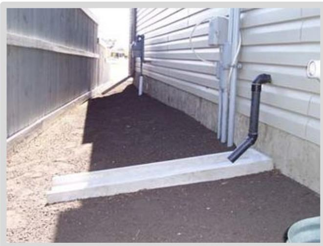
Figure 16 – Splash pad at downspout discharge can prevent erosion. Source: The City of Edmonton Residential Lot Grading Guide
