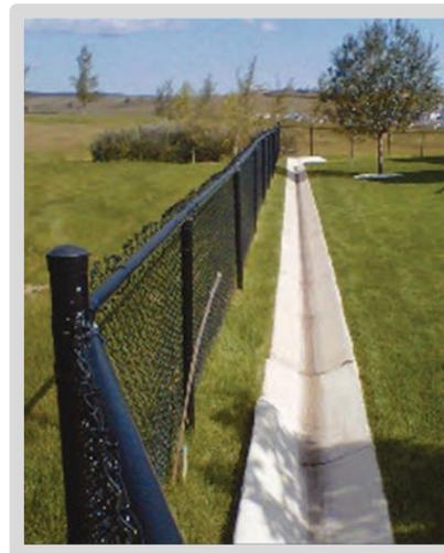
*Minimum 0.6% Slope in Concrete Swales. Source: The City of Calgary*
