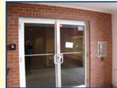
This entry is designed with an anti-jimmying plate on the door, an outside intercom, a security camera and glass security doors which provides the tenants with access control and good surveillance. This also increases security at the site and reduces fear for tenants.
