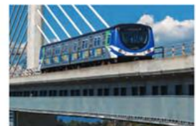
Automated People Mover (APM) SkyTrain, Vancouver
