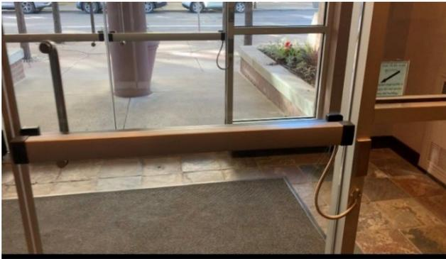
Figure 2: Panic hardware tied into the magnetic lock
