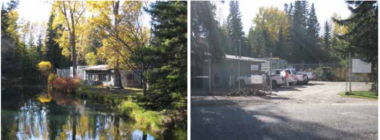
Parks maintenance facility at entrance to Bowness Park.
