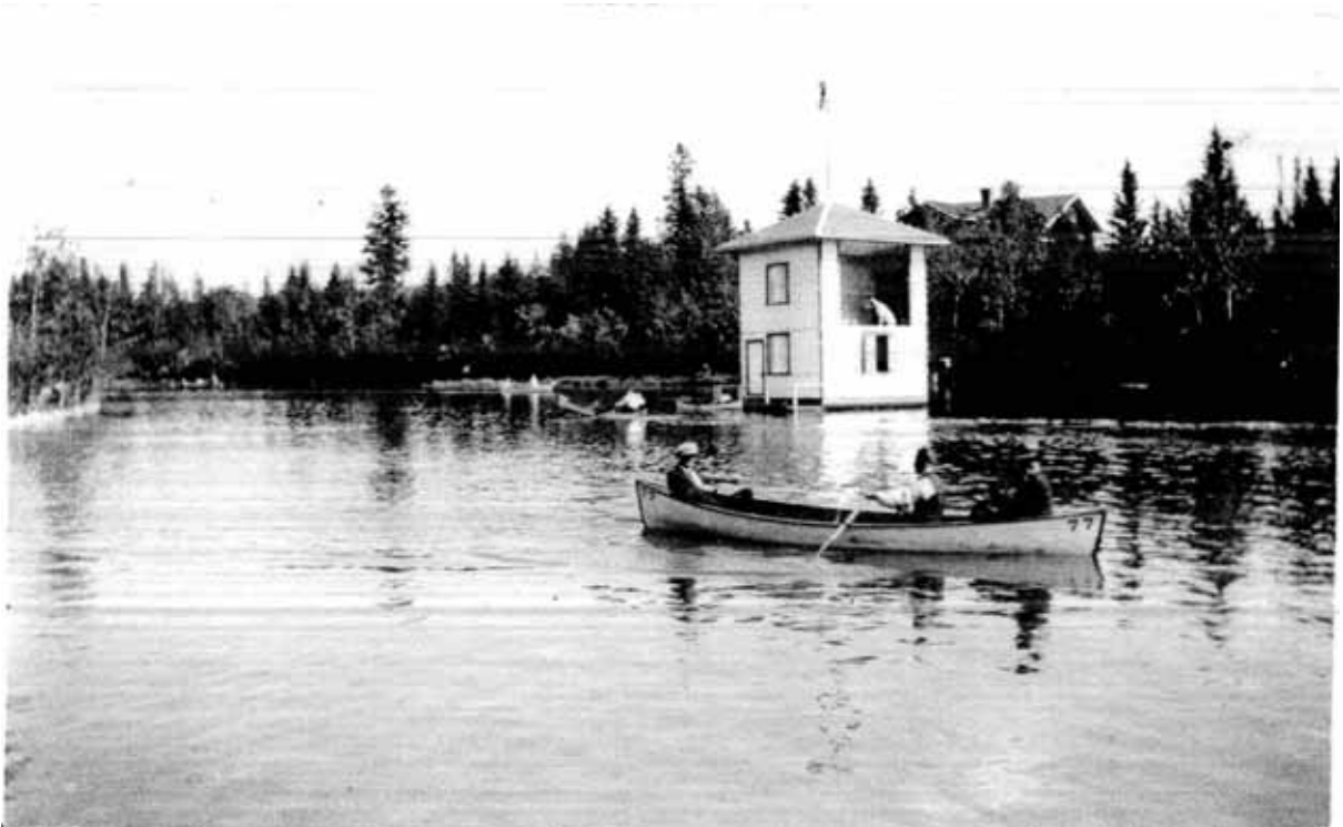
Former 'Orthophonic' structure at Bowness Park Lagoon.
