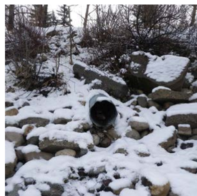
Images depicting the slope dewatering system on the escarpment at the south end of the study area
