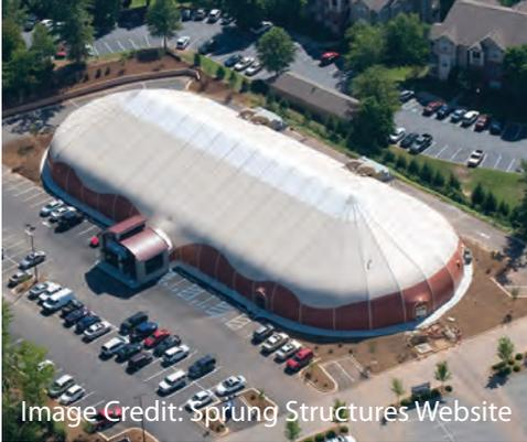
A fabric covered steel frame (e.g. sprung) structure is another indoor option, however, the span of these buildings is generally limited to approximately 60 m in width. These buildings are generally less expensive than a pre-engineered building.
