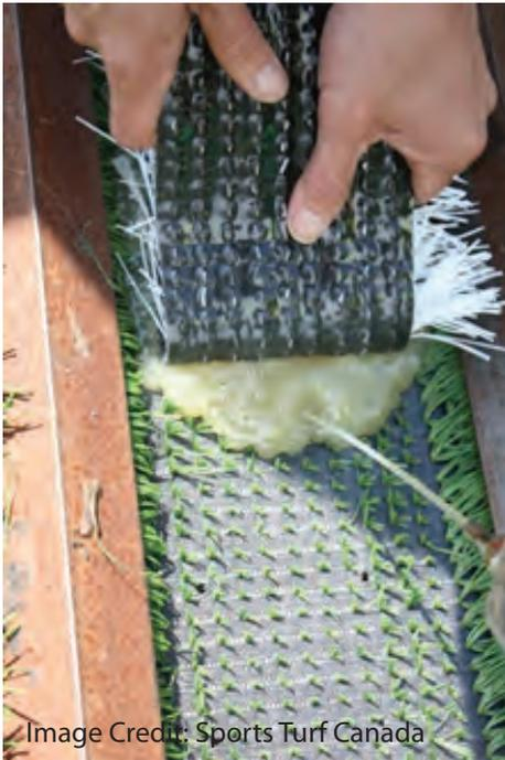
Figure 5.22- Seam that Needs Repair
