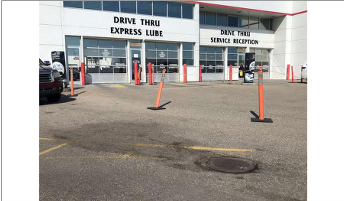
**Photo 35** Pavement staining leading to a paved drainage area on the Country Hills Toyota dealership property.
