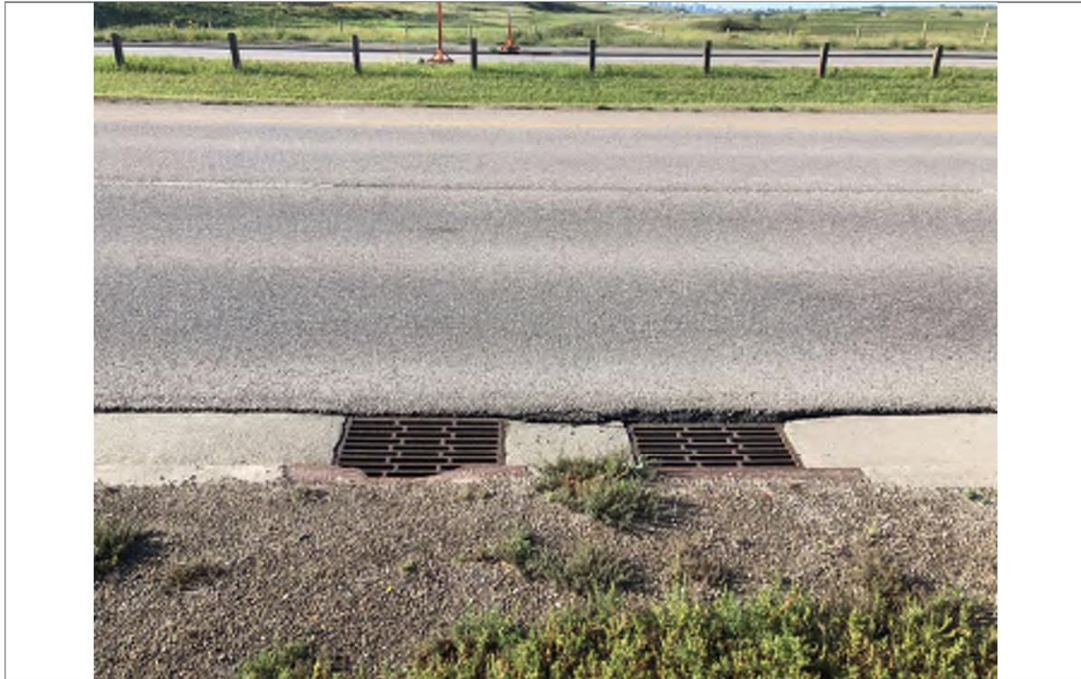
**Photo 23** An example of the curbside paved drainage grates and catch basins along CHB.
