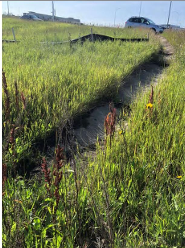
**Photo 16** Stormwater drainage pathway for the northern side of CHB, leads to stormwater outfall “N 42”.
