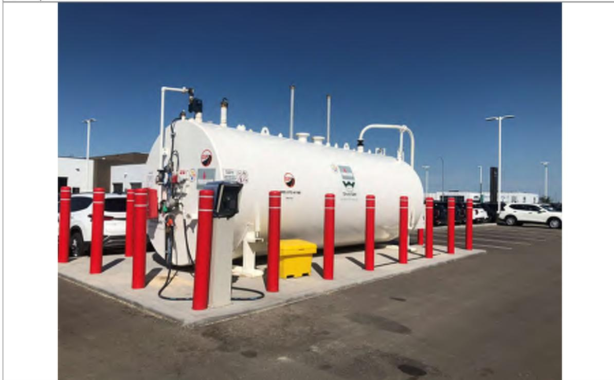
**Photo 44** Storage tank located on the western side of the Country Hills Nissan dealership property, as well as adjacent minor pavement staining.
