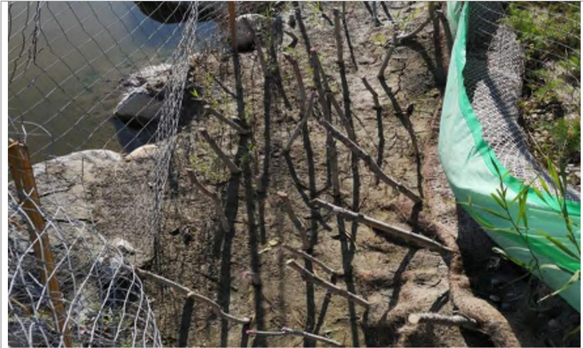
**Plate 11** Willow sp. bank stabilization, Nose Creek, Outfall #42 (SE 26-25-01 W5M; approximately 11U 707428E/ 5671175N) (August 15, 2019).
