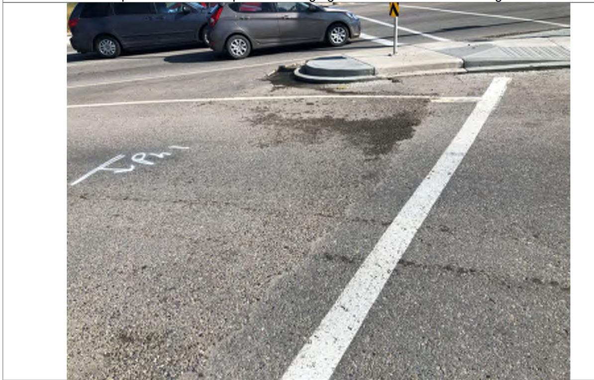
**Photo 24** Pavement staining at the 14 Street NE and CHB intersection.
