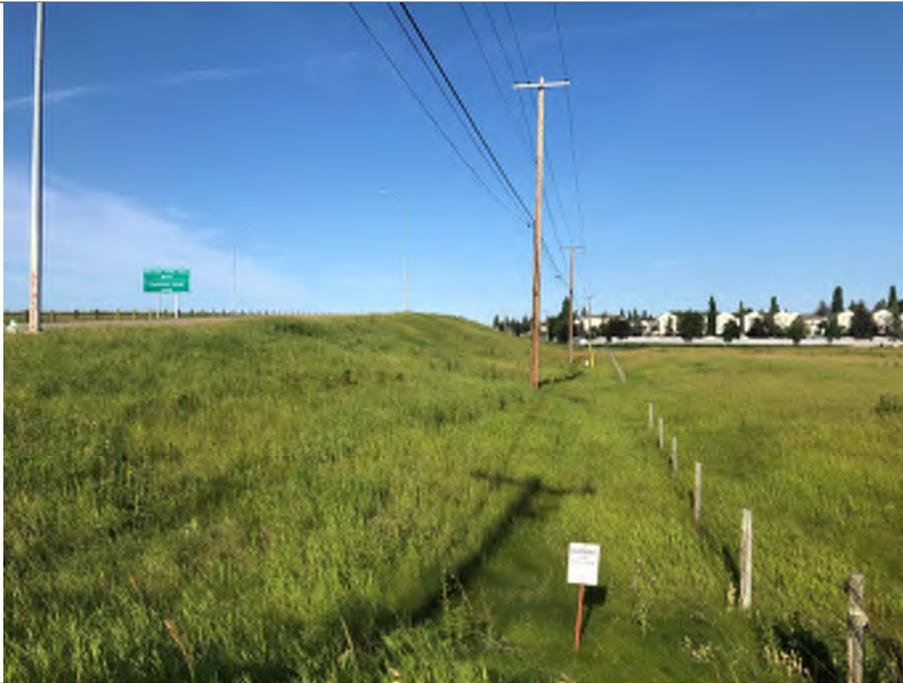
**Photo 7** Minor overhead transmission lines (running east-west), underground natural gas pipeline (running east-west) warning sign; western view, taken from the north side of CHB from the west end of CHB
