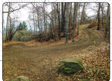
SHARP SWITCHBACK WITH STEEP SLOPE BEFORE AND REDUCED VISIBILITY (AS A RESULT OF DENSE VEGETATION AND TREES)
