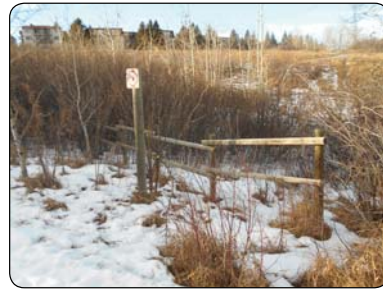
EXISTING WOODEN RAILING & SIGNAGE
