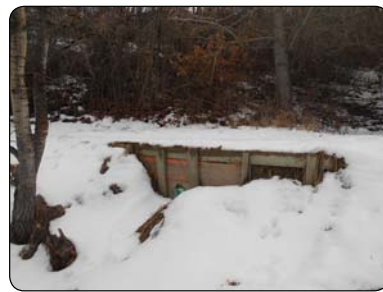
EXISTING CULVERT & WOODEN RETAINING WALL
