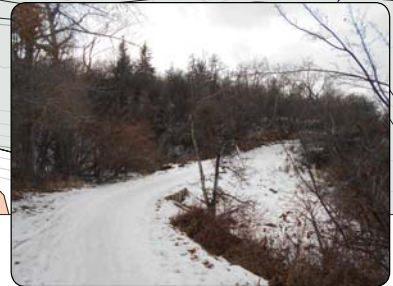
SHARP TURN WITH STEEP SLOPE BEFORE AND STEEP SHOULDER WITH NO GUARDRAIL
