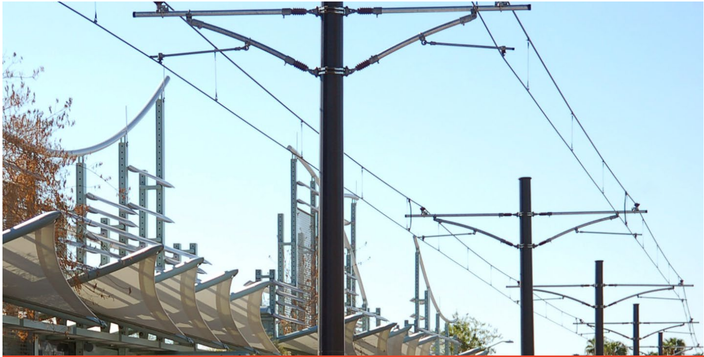
W1 Aesthetically Treated Simple Catenary Wire with Low Profile (SCAT-LP)
