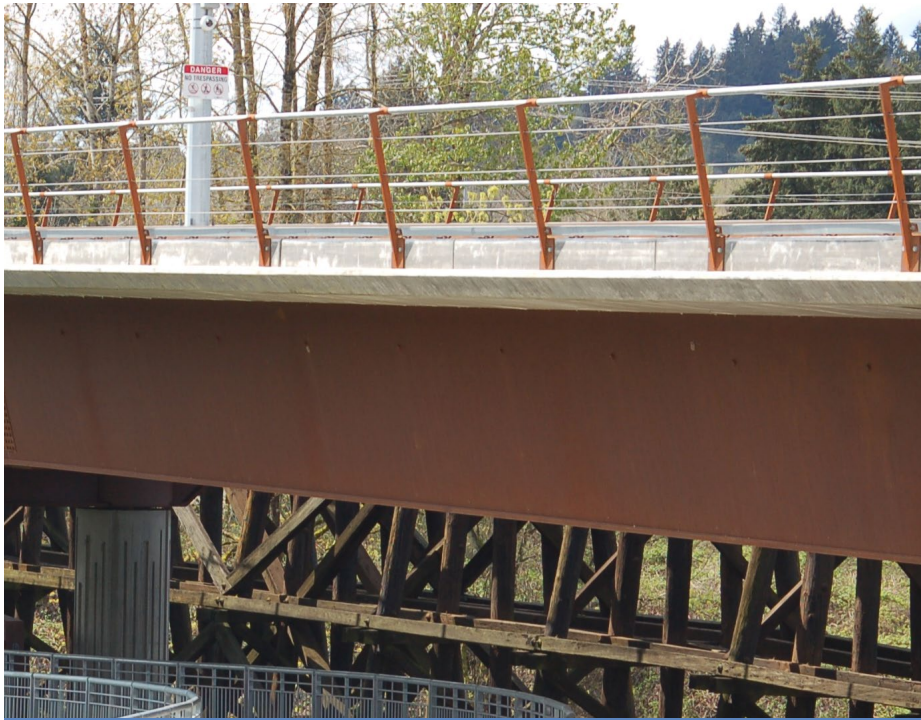
R7 Safety railing: steel stanchions and cable guideway
