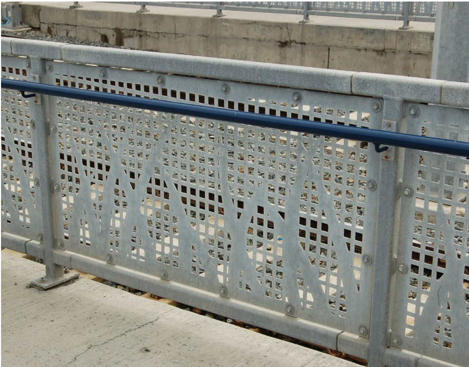
R5 Station railing: galvanised metal punched or cut panel
