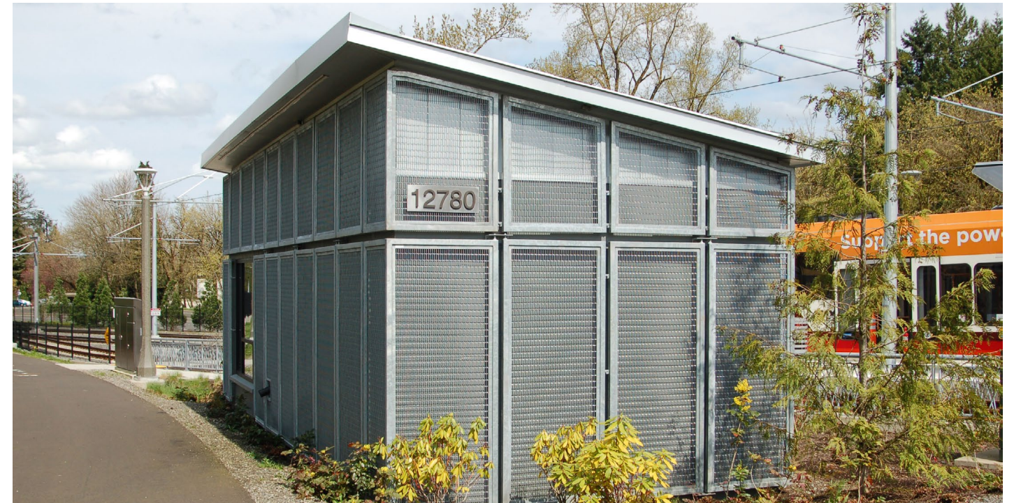
SYS2 CMU with metal mesh cladding
