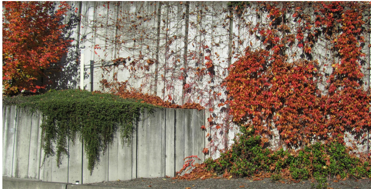
RW1 Retaining walls: cast-in-place, form-liner
