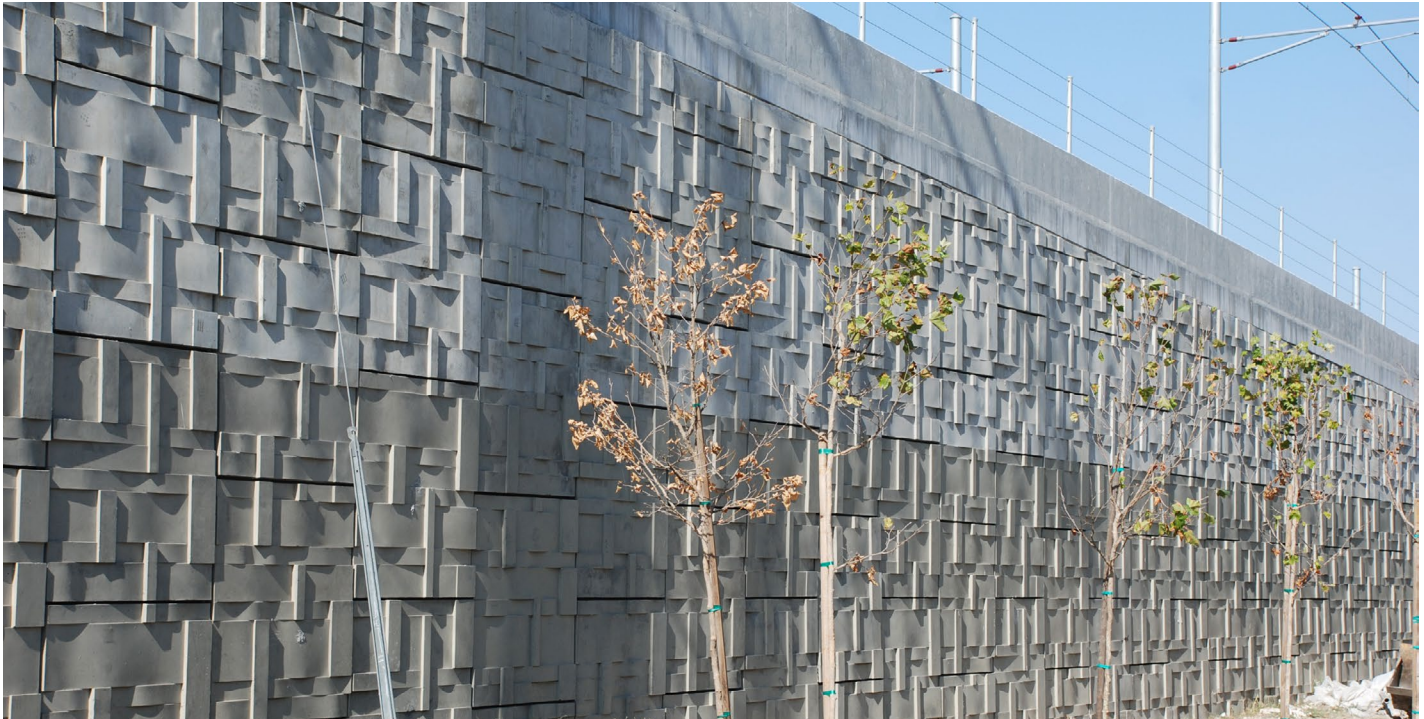
RW2 Retaining walls: MSE- large cell, form-liner
