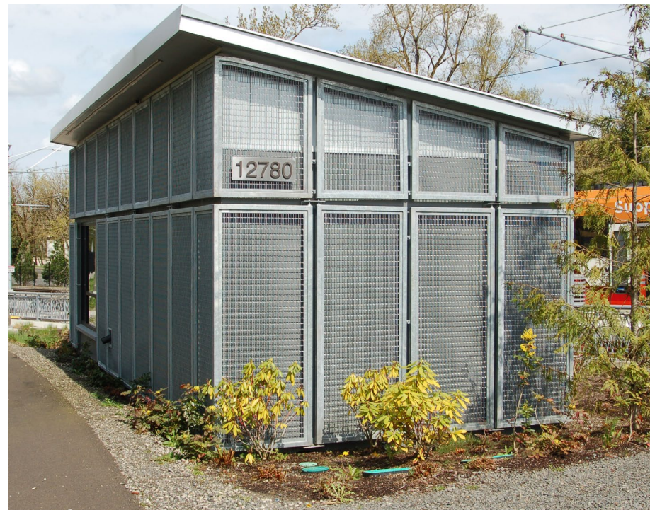
SYS2 CMU with metal mesh cladding
