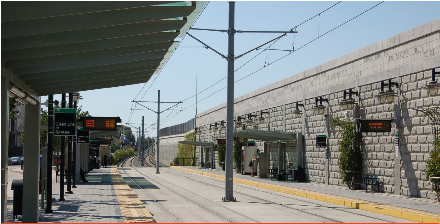
PL1 Pole: round/beveled galvanised steel poles-single use
