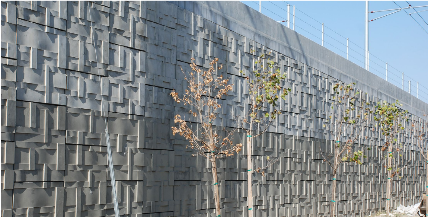
RW2 Retaining walls: MSE- large cell, form-liner
