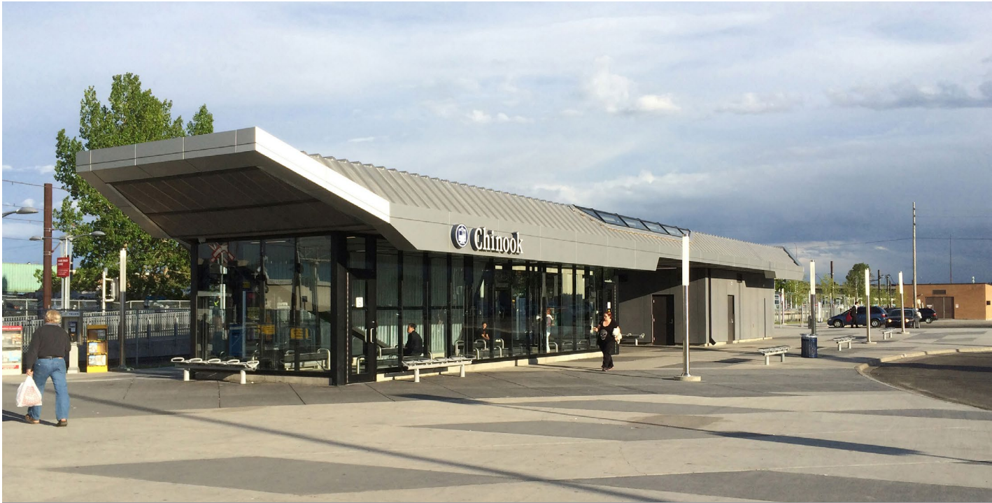
SYS6 Operator break building (OBB): metal cladding, roofing, glass curtain wall
