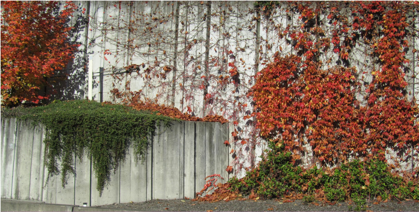
RW1 Retaining walls: cast-in-place, form-liner
