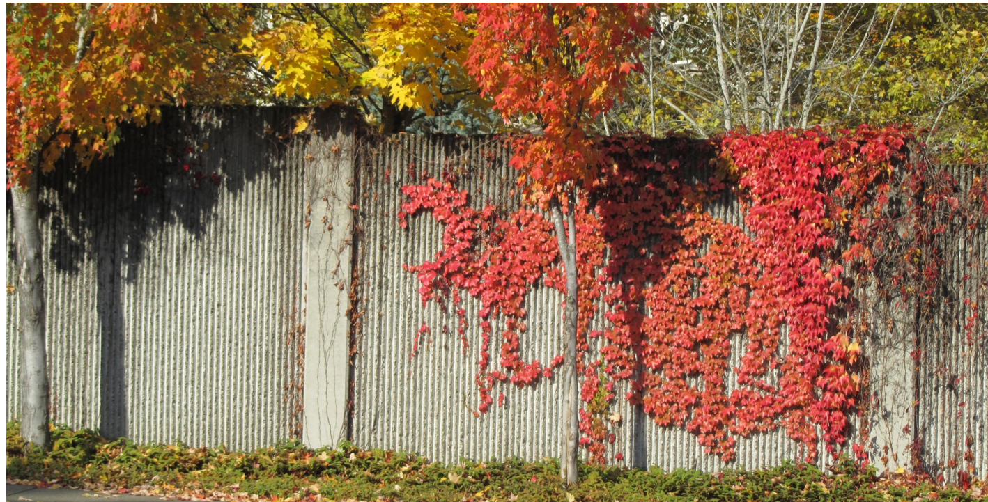
RW5 Sound attenuation walls: precast concrete formliner
