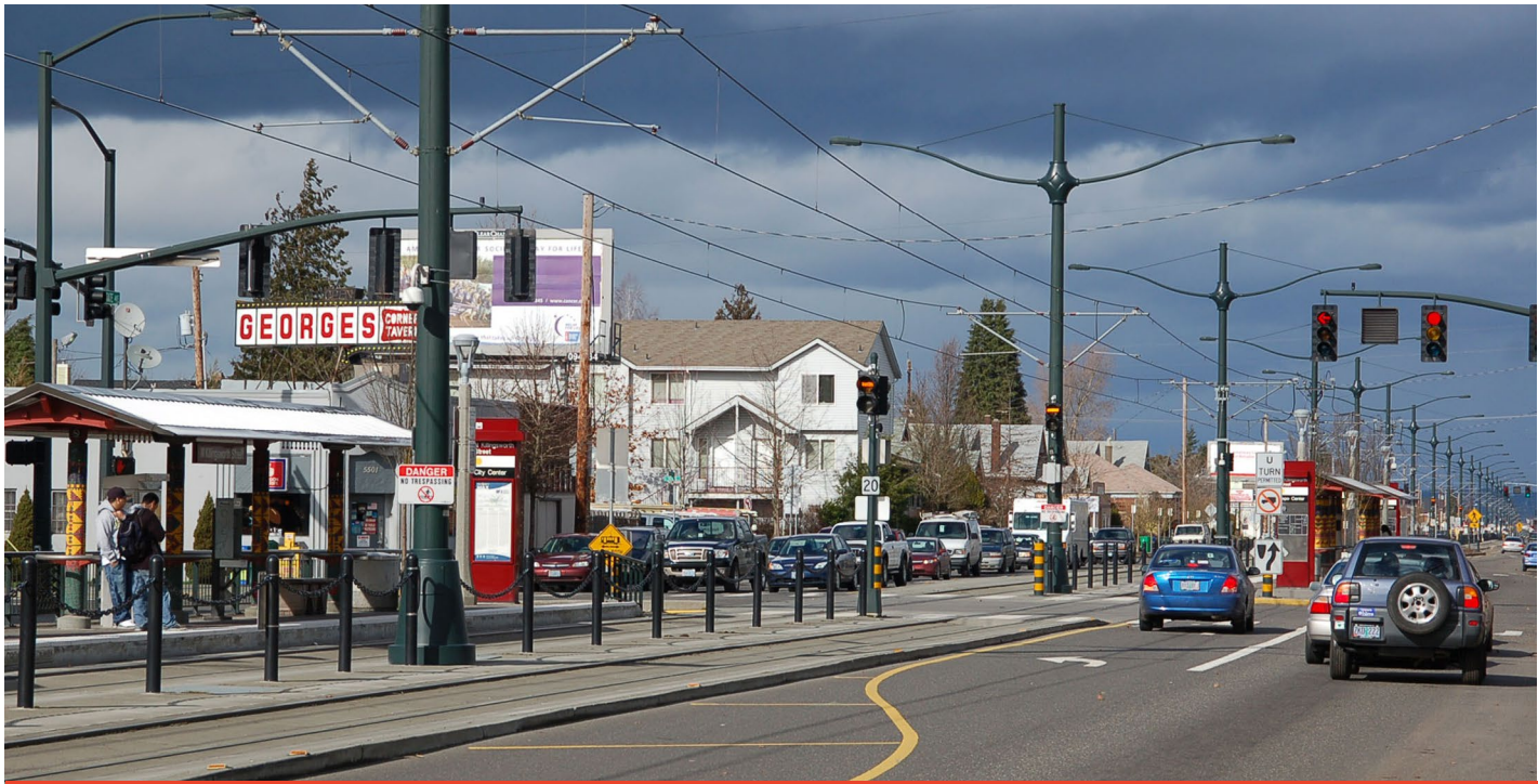
PL2 Pole: round galvanised steel poles: shared use with street lights, traffic, pedestrian and cycle signals
