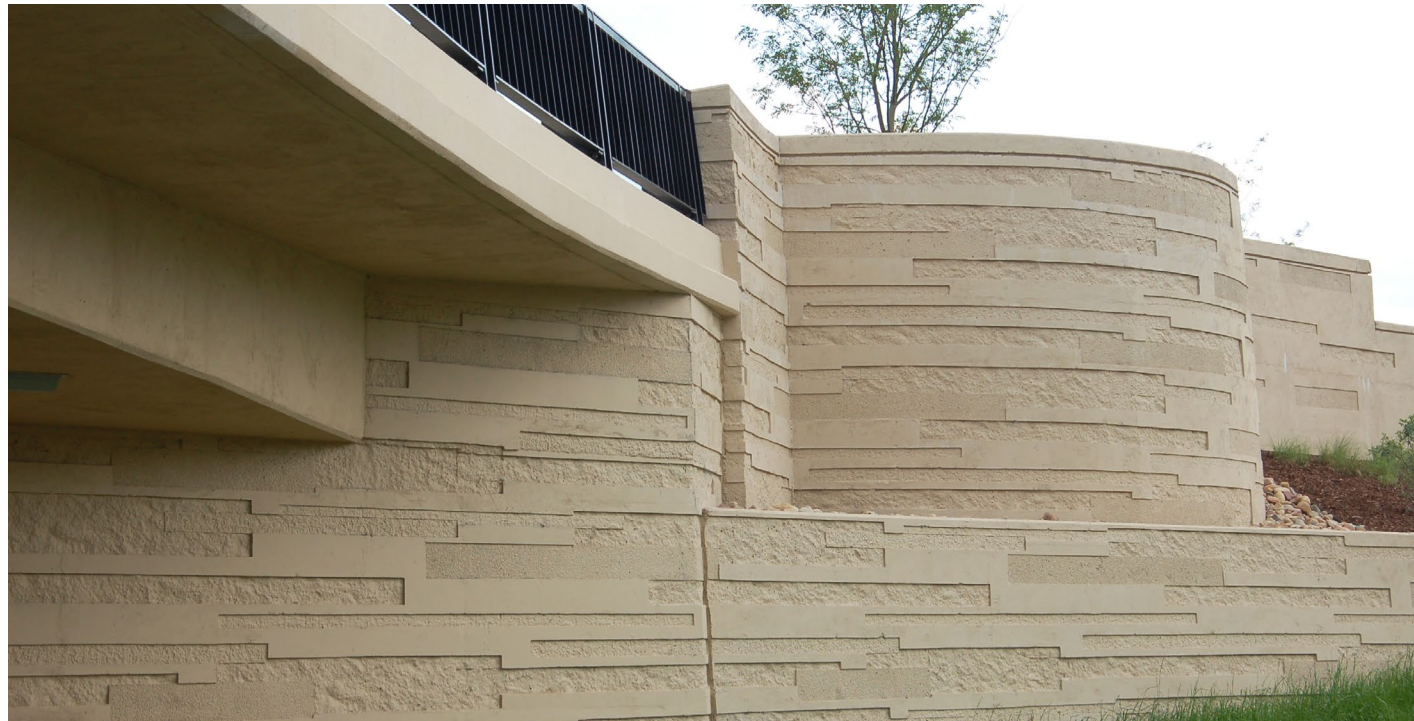
RW7 Screening walls: pre-cast concrete - formliner
