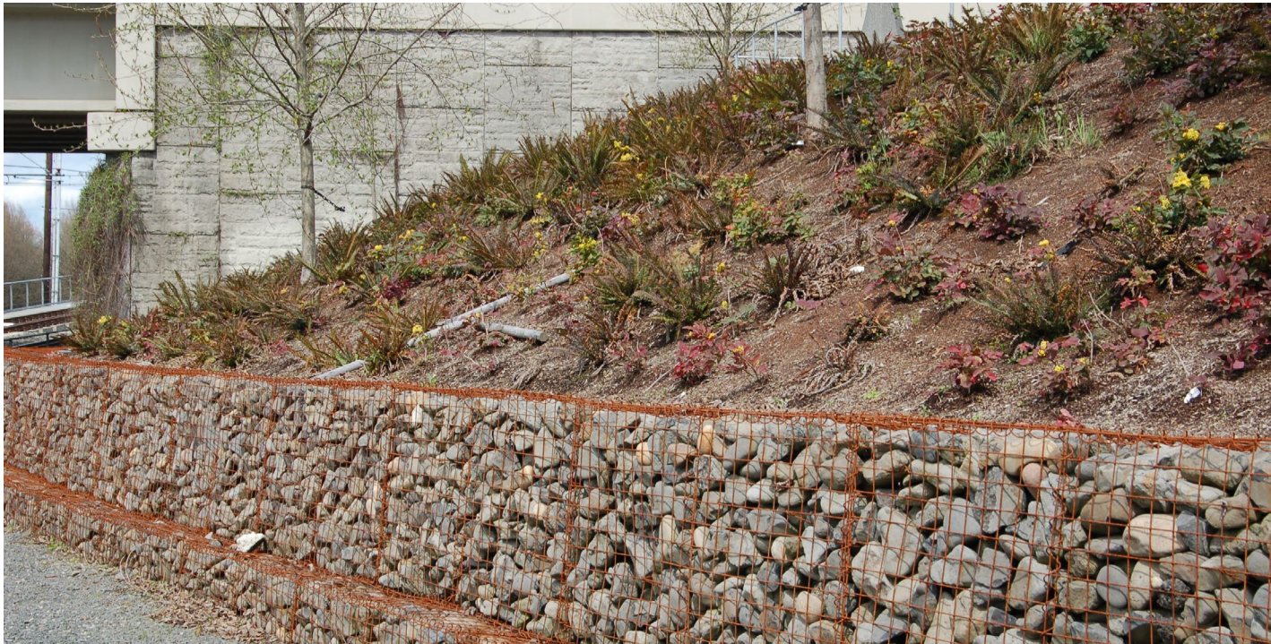
RW4 Retaining walls: gabion, rock or glass aggregate
