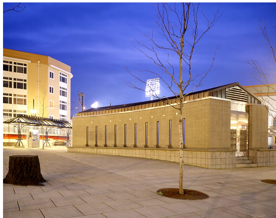
SYS4 Concrete base, CMU and glass block walls, metal roof
