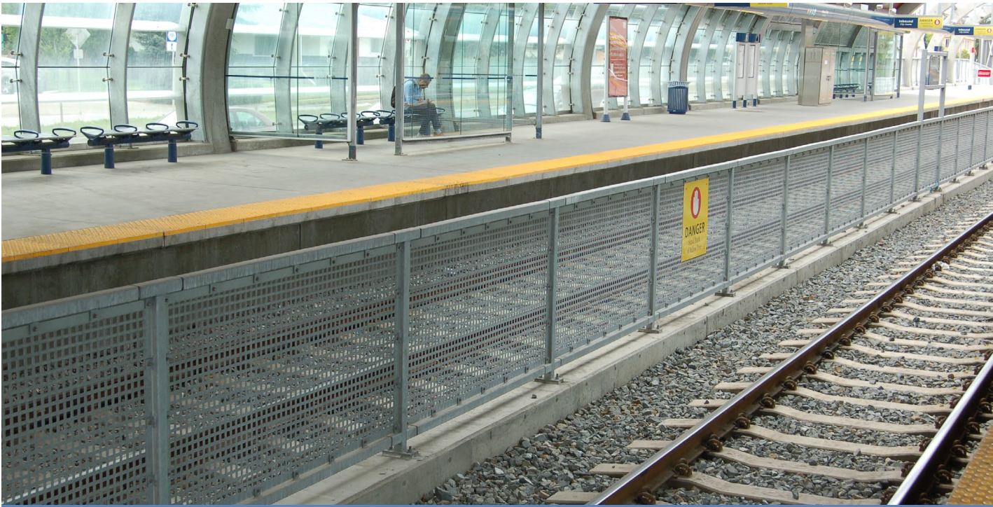
IT2 Inter-track barrier: galvanised metal punched or cut panel
