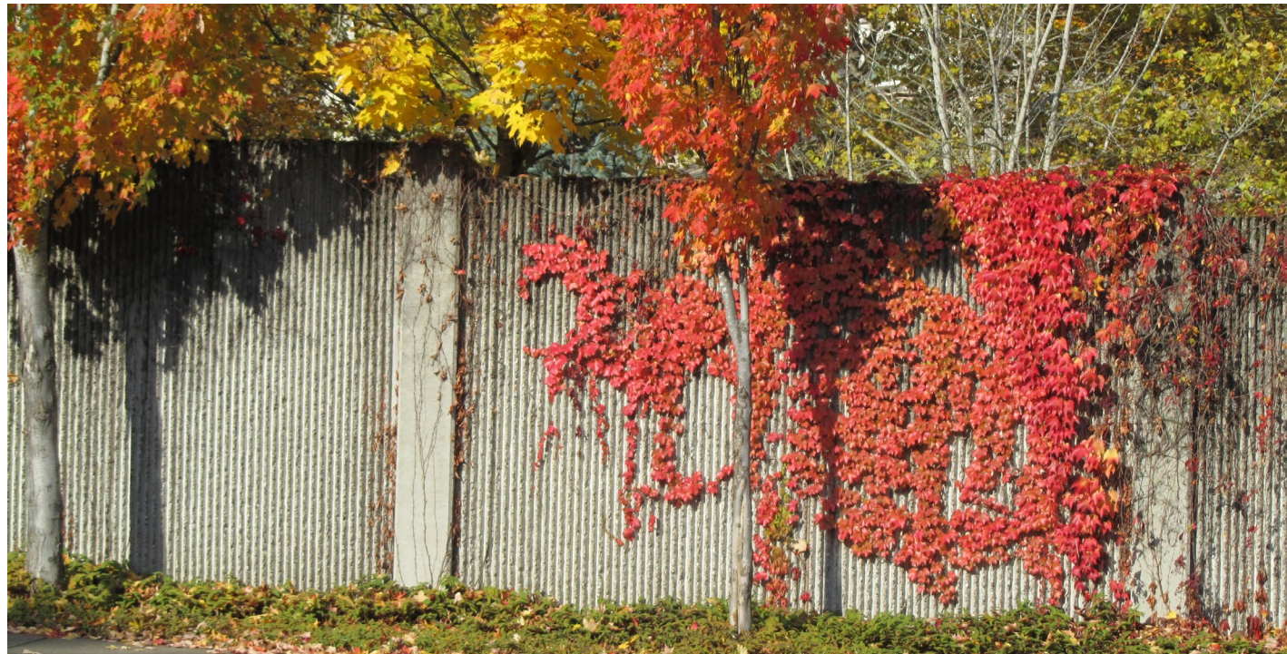
RW5 Sound attenuation walls: precast concrete formliner
