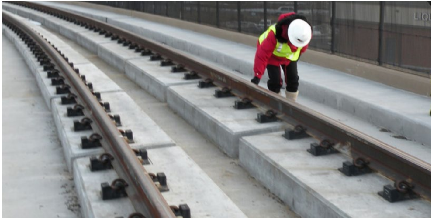
TW2 Direct fixation track
