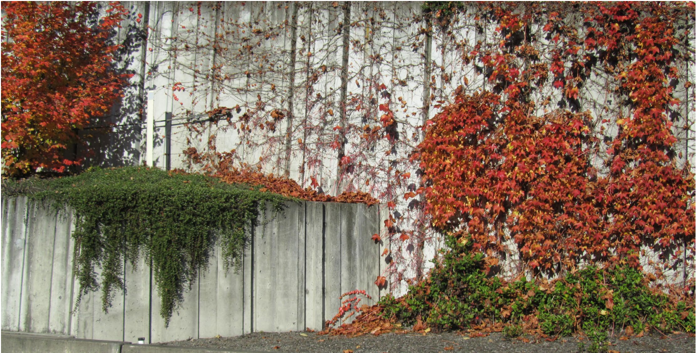
RW1 Retaining walls: cast-in-place, form-liner
