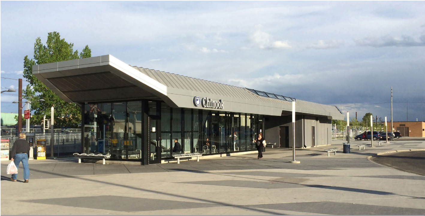
SYS6 Operator break building (OBB): metal cladding, roofing, glass curtain wall
