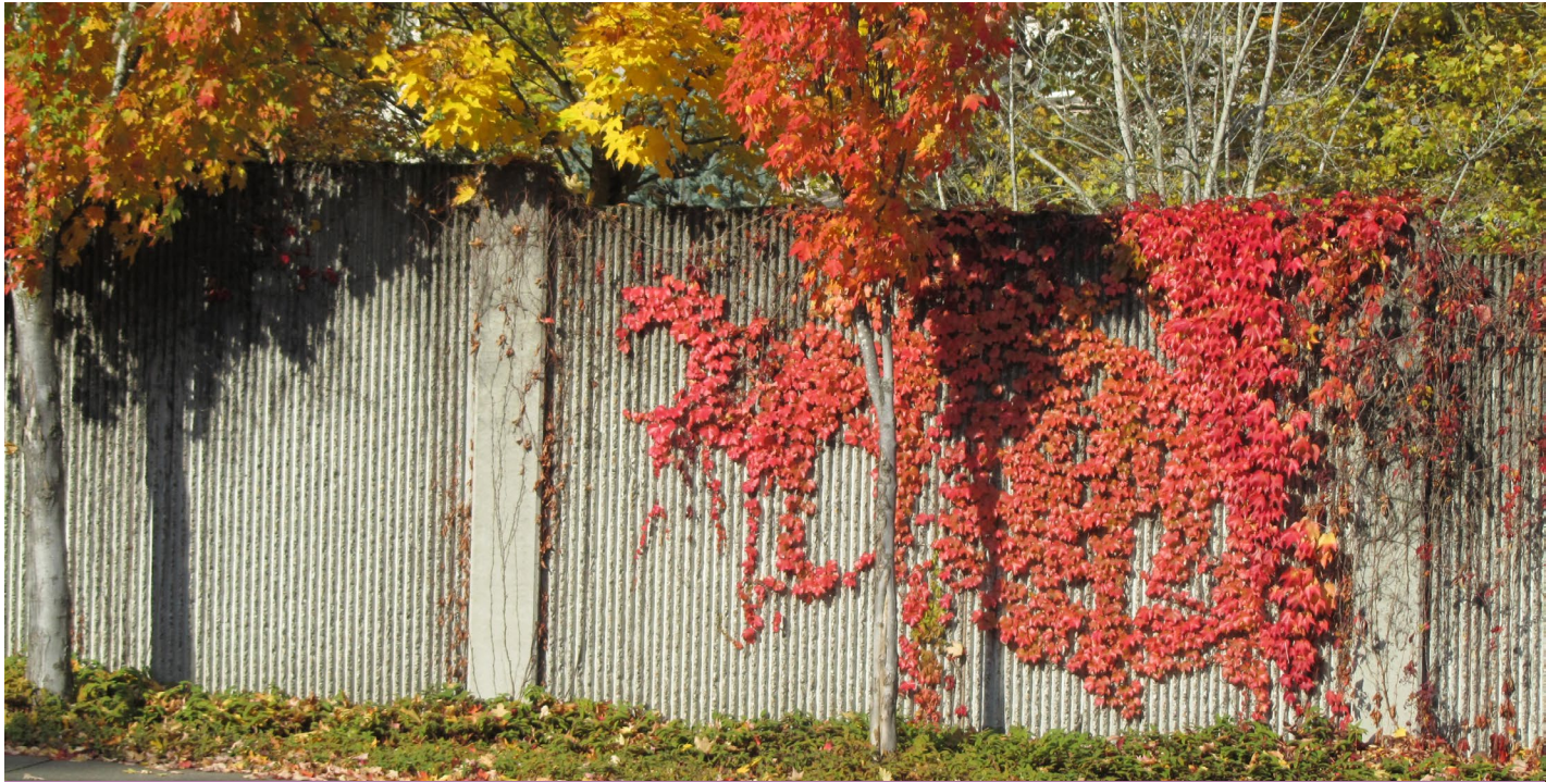
RW5 Sound attenuation walls: precast concrete formliner
