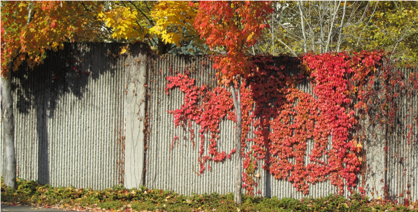
RW5 Sound attenuation walls: precast concrete formliner
