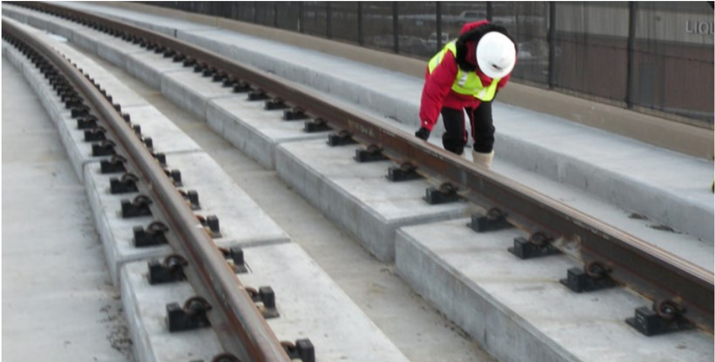
TW2 Direct fixation track
