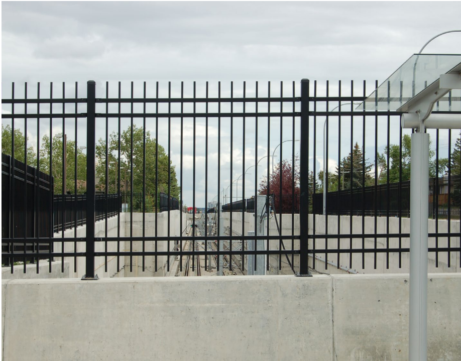
R1 Station railing: painted or coated metal picket
