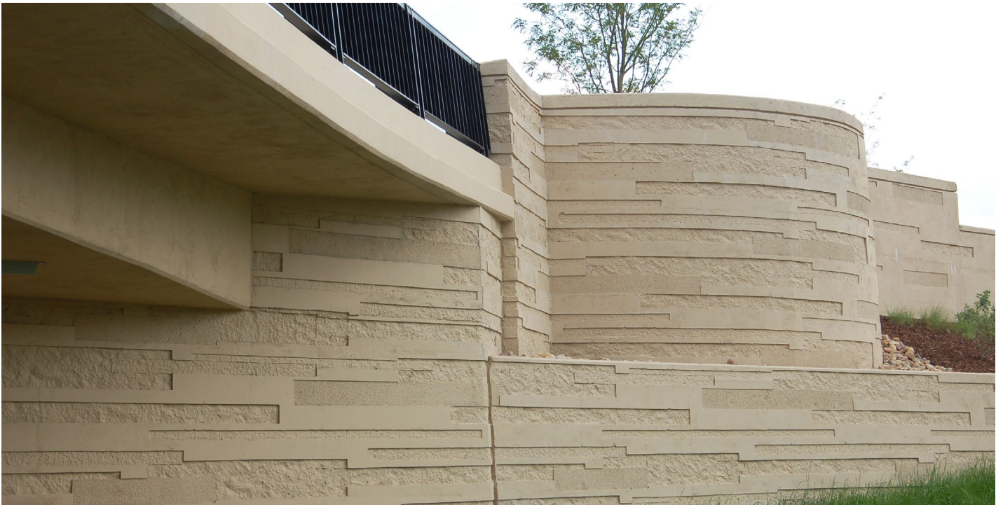
RW7 Screening walls: pre-cast concrete - formliner
