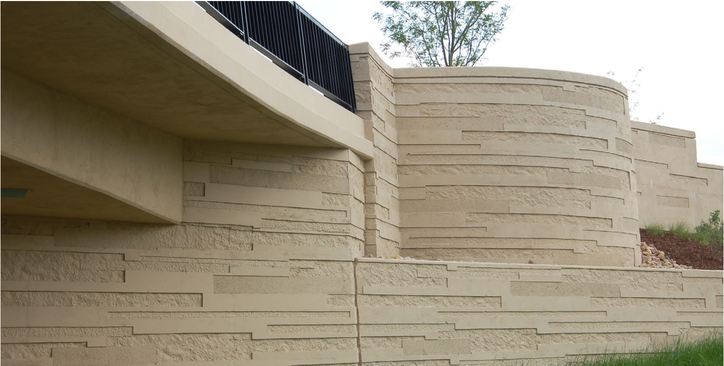
RW7 Screening walls: pre-cast concrete - formliner
