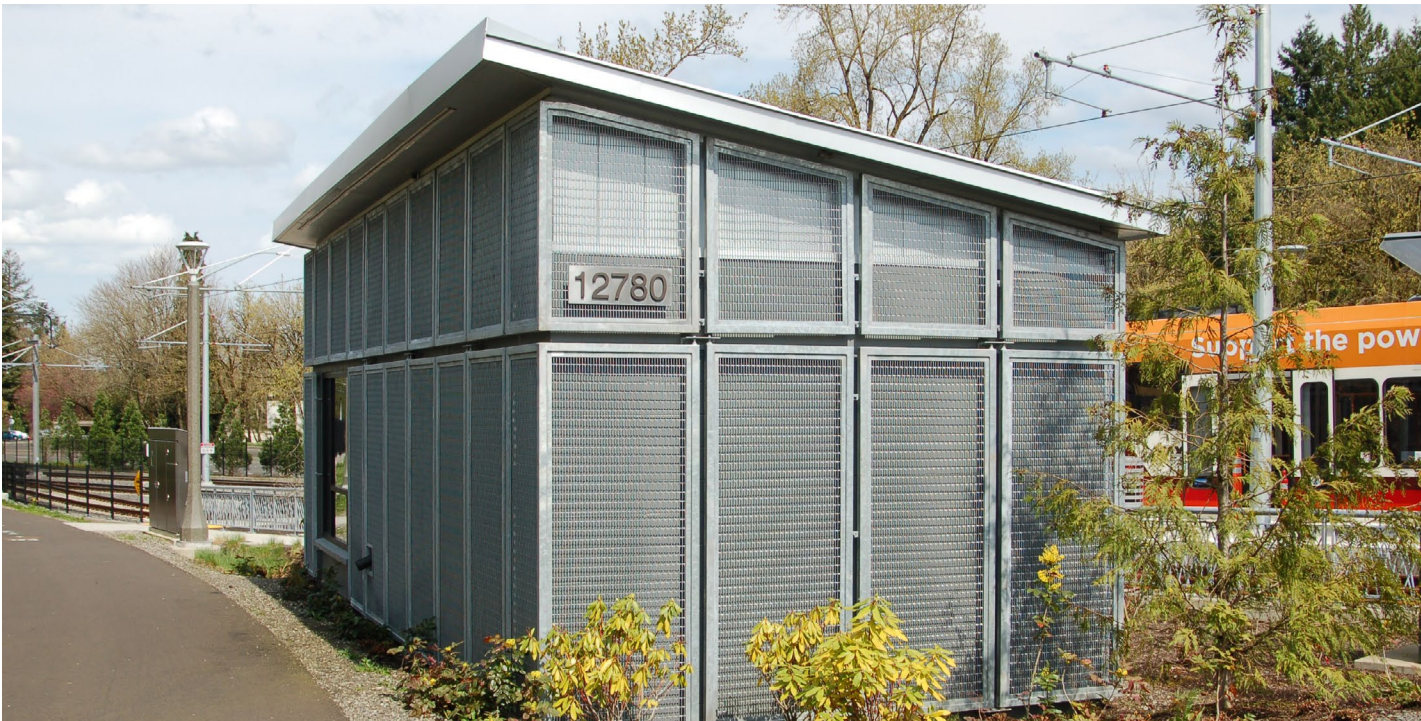
SYS2 CMU with metal mesh cladding
