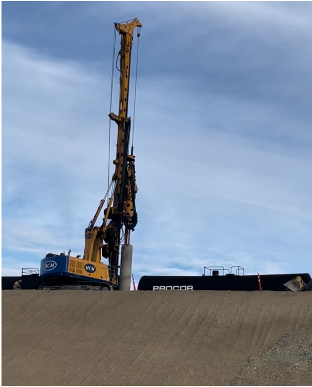
Looking at the Secant Pile Wall installation works on top of the newly constructed 78 Avenue diversion track embankment.
