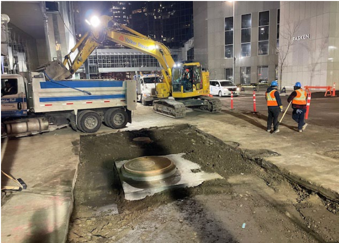
Looking east at CHDI work in Downtown (6 Avenue S.E.).
