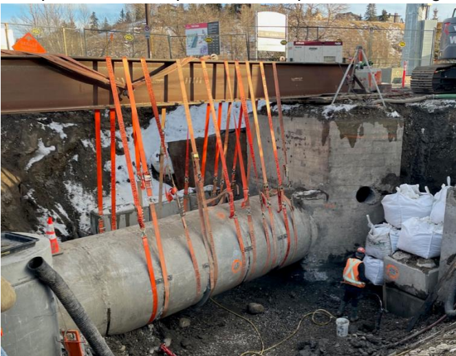
Looking Southeast at manhole installation work at 12 Avenue & 6 Street SE
