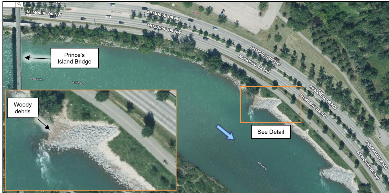
Figure K Woody Debris Downstream of Project (2022 Imagery from City of Calgary)
