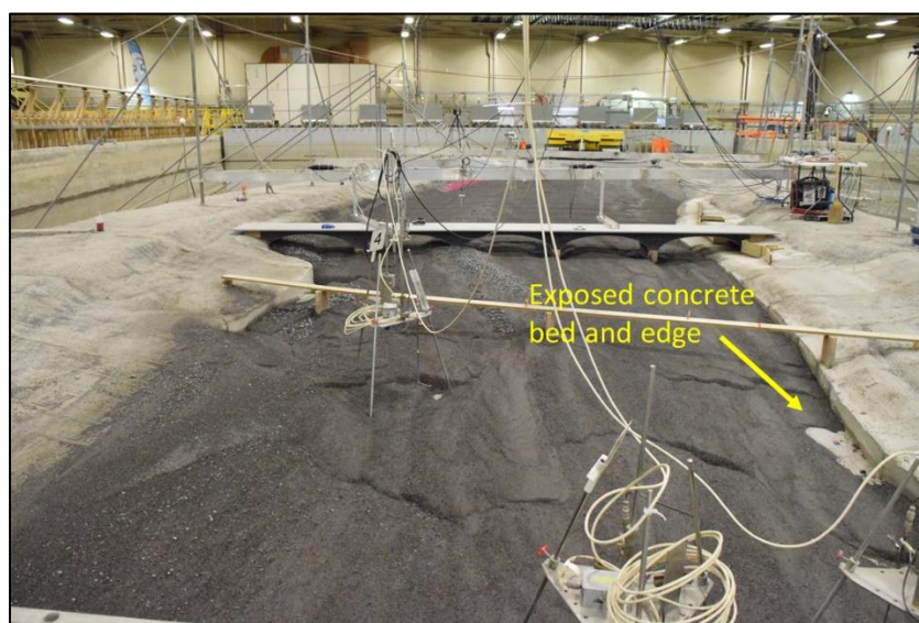
Figure 111. Example of scour exposing the concrete bed and the edge of the concrete bed.
