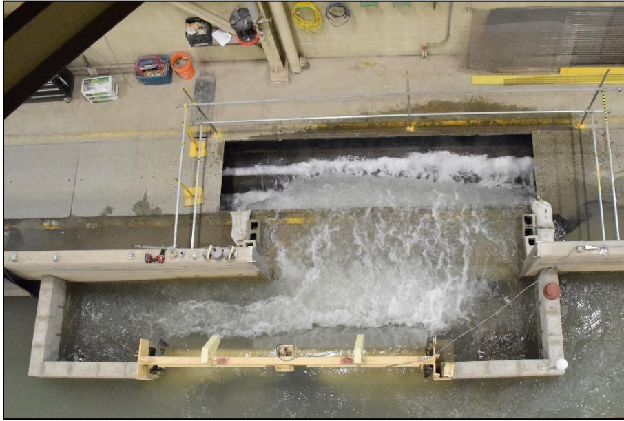
Figure 22. Flow spilling over the control weir into the reservoir sump (photo taken from above).
