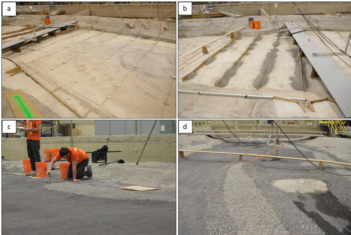
Figure 16. Various stages of the mobile bed construction; a) shows pads installed and levelled on top of the concrete bed, b) shows fiberboard templates installed on top of the levelled pads and prepared for backfilling, c) shows an example of bioengineering stone being installed by hand near Poppy Plaza, and d) shows a portion of the final mobile bed for conceptual design #2 looking downstream from Louise Bridge; riprap material (with voids filled with river sediment) is visible on the edges of the main bar, bioengineering stone is visible on top of the main bar, and transition cobble is visible behind the right (south) pier of the LRT bridge.
