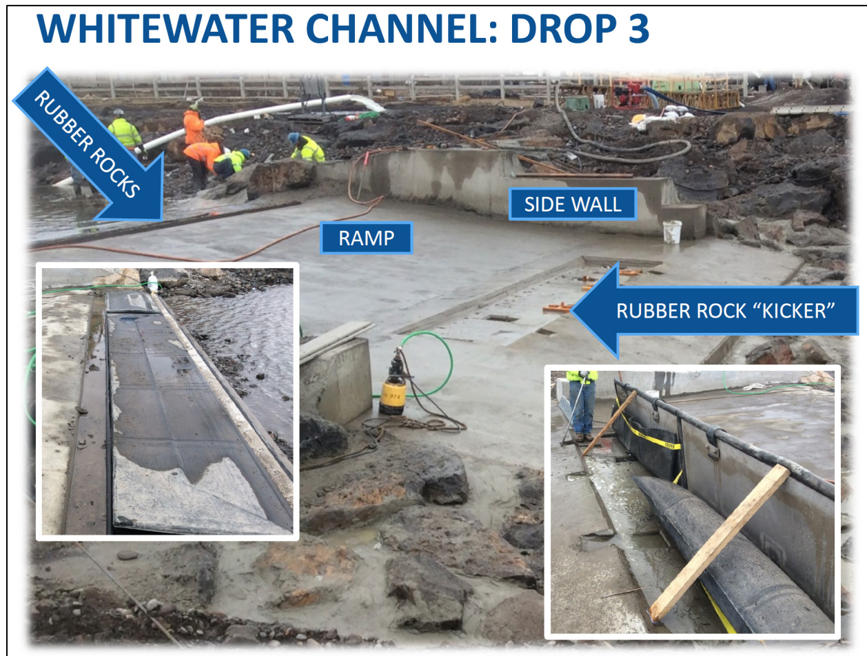
Figure 19: Installation of the pneumatic kickers in Bend, USA.
