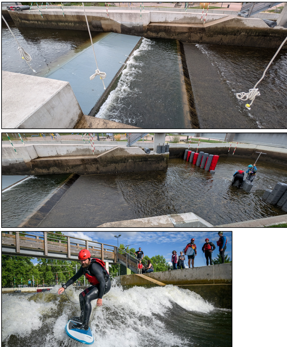
Figure 64: Flap gate with downslope wave in Epinal, France.
