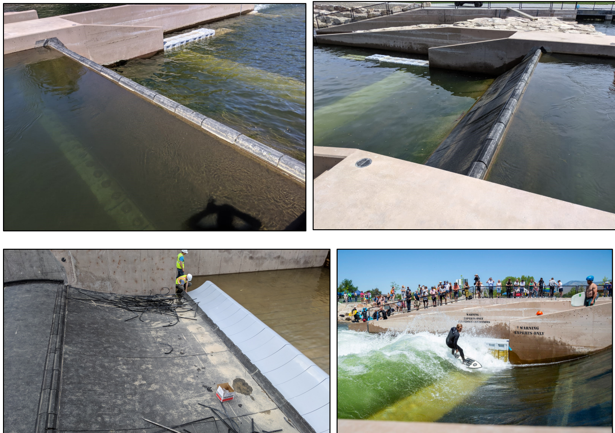
Figure 26: Boise Phase 2 flap gate with downslope forming a wave.
