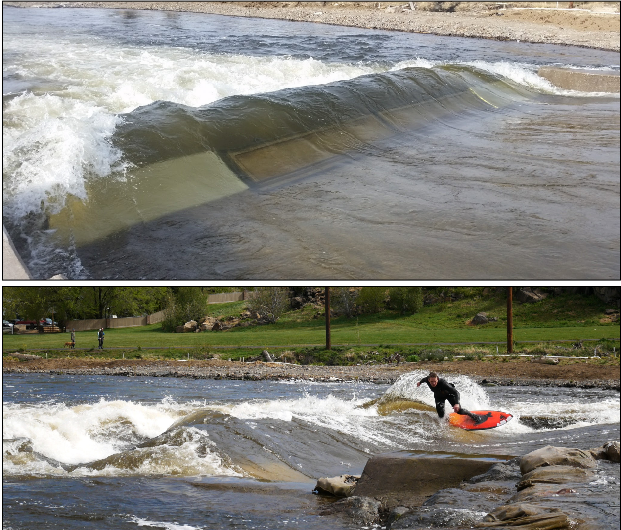
Figure 18: Pneumatic kickers creating a good river wave in Bend, Oregon, USA.
