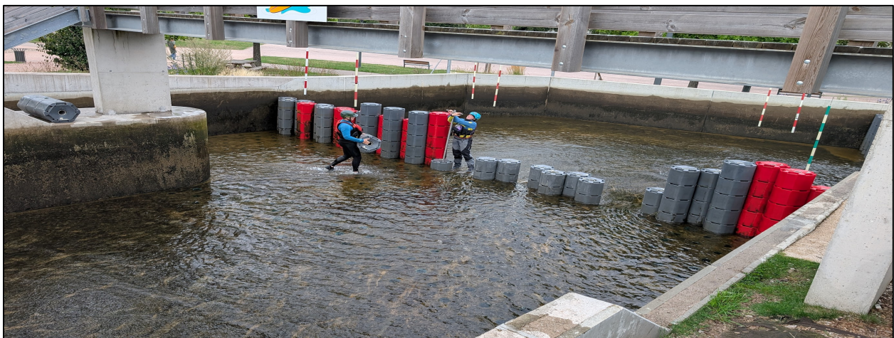
Figure 47: Adjustable walls in a whitewater park in Epinal, France.
