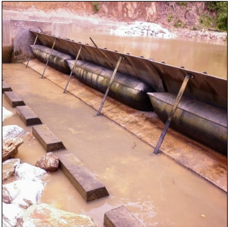
Figure 22: 1.5m high Obermeyer pneumatic gate installed.
