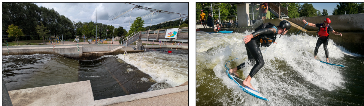
Figure 25: Epinal, France, raised flap gate with downslope making a wave.
