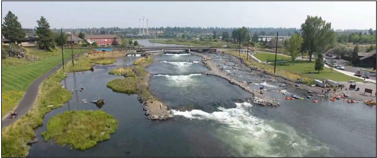
Figure 62: Bend – Habitat on left, Waves in middle, Tuber Passage on right. Replaced hazardous dam.
