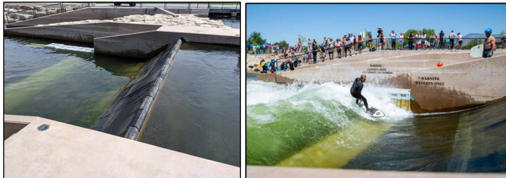
Figure 23: Boise, USA, flap gate with downslope blocking flow and making wave
