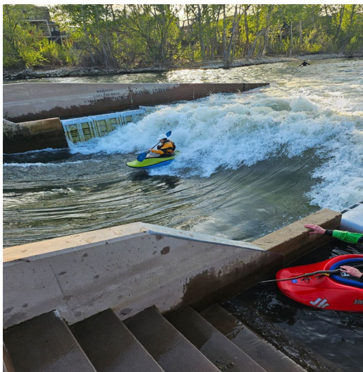
Figure 58: Adjustable wall at Boise, USA
