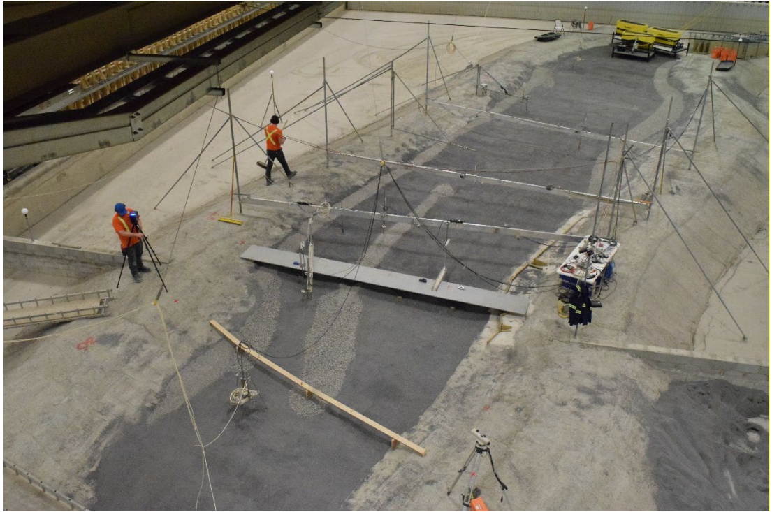
Figure 35: Physical modelling trial run setup. Proposed riprap stabilization is in place along the south slopes and the realigned gravel bar.
