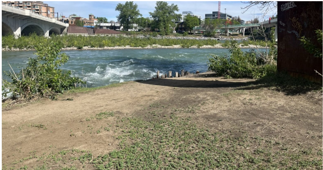
Figure 26: Poor bank condition and trampled vegetation at the existing wave location
