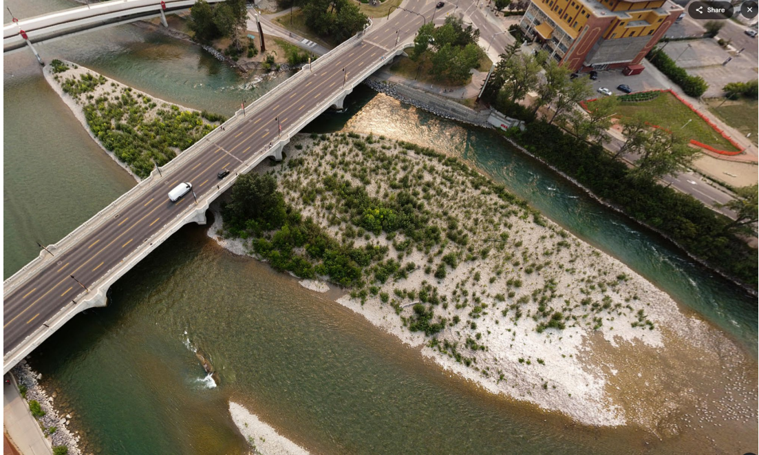
Figure 4: Drone photograph of Louise gravel bar, facing south towards downtown Calgary. Note vast extents and large amounts of vegetation
