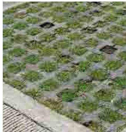
Permeable pavers - turf grid
