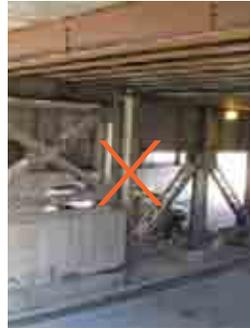
5. Existing pipes and cables underneath the superstructure should be either encased or visibly enhanced through bright coloring.
