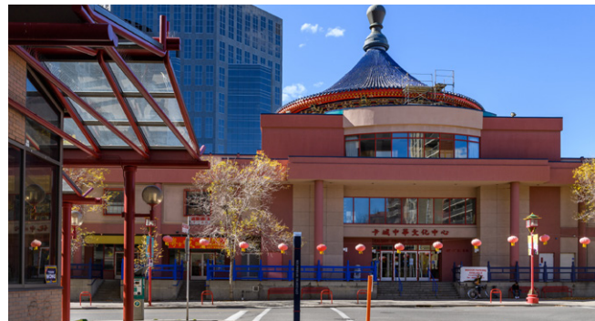
Calgary Chinese Cultural Centre, constructed in 1992
