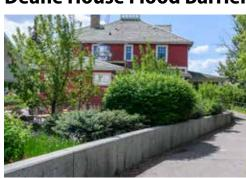
Stops high flows from the Elbow River flooding into Inglewood
