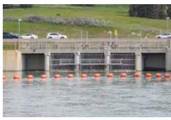
Improvements to the Bow River bank downstream of sluice gates to permit opengate conditions during high water events.
