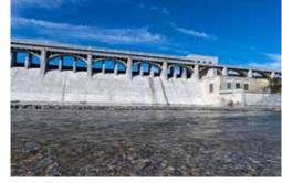
A new steel gate and hoist system to capture and temporarily hold more floodwater in the reservoir during an emergency. 21 new steel gates span the length of the dam
