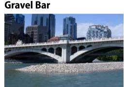
Gravel bars that have the potential to become vegetated can block flow during a flood.
