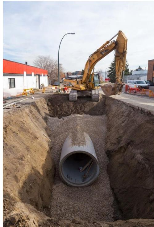
**Stormwater management** in the established area is a significant challenge for developers and The City. Many of the public stormwater management systems in the established area were built to earlier standards and have lower capacity. Combined with changing weather patterns, and increased impermeability as a result of redevelopment, flood risks are increased in these areas.
