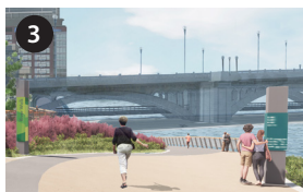
3 Centre St. Pedestrian Ramp Upgrades Spring 2022
