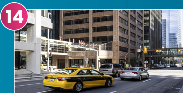
14 510 5th 510 5 Street S.W. Bluevale Capital Group 128 Units 112,000 sq. ft. Converted
