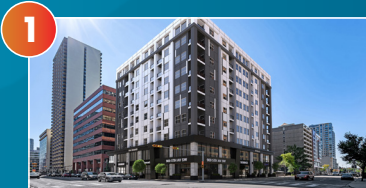
1 THE CORNERSTONE 909 5 Avenue S.W. Peoplefirst Developments 112 Units 111,000 sq. ft. Converted
