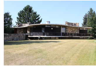
Blum Residence (built 1963) Municipal Historic Resource Designated November 2018
