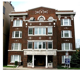
Lorraine Apartments (built 1912-1913) Conservation Grant Recipient
